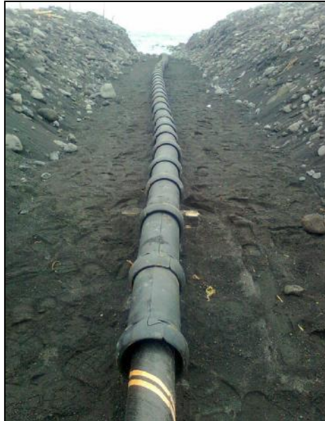
Figure 40: Example Split Pipe Installation
