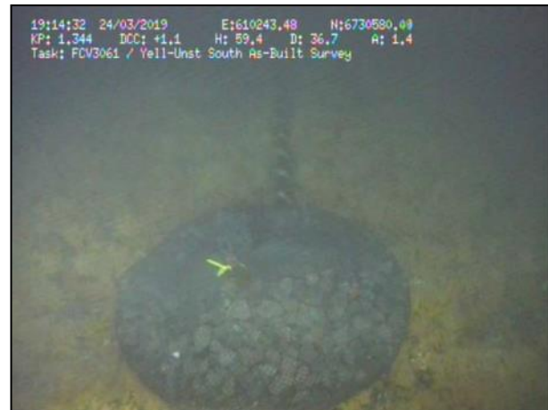
Figure 309: Rock Bag in Position Subsea
