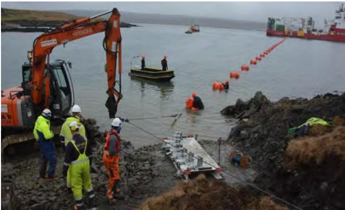
Figure 11: Example of the Beach Quadrant Layout during pull-in
