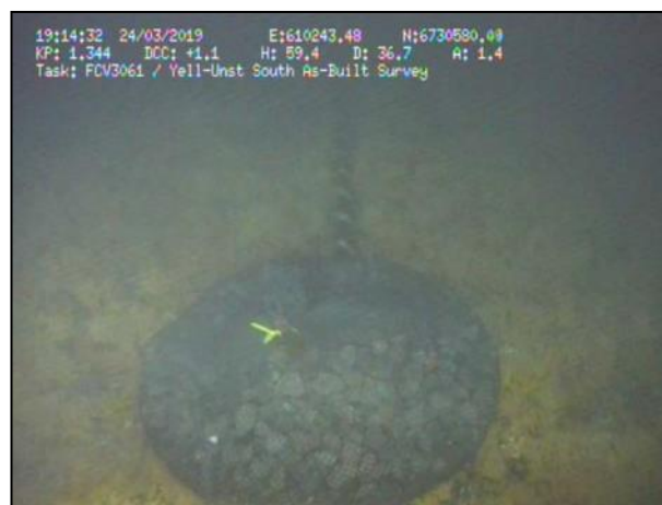
Figure 298: Rock Bag in Position Subsea
