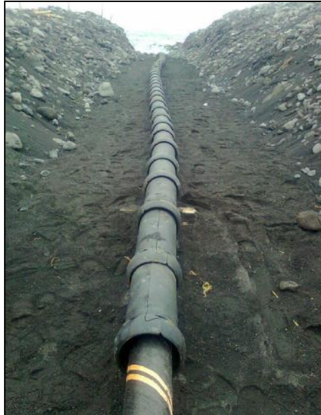
Figure 41: Example Split Pipe Installation
