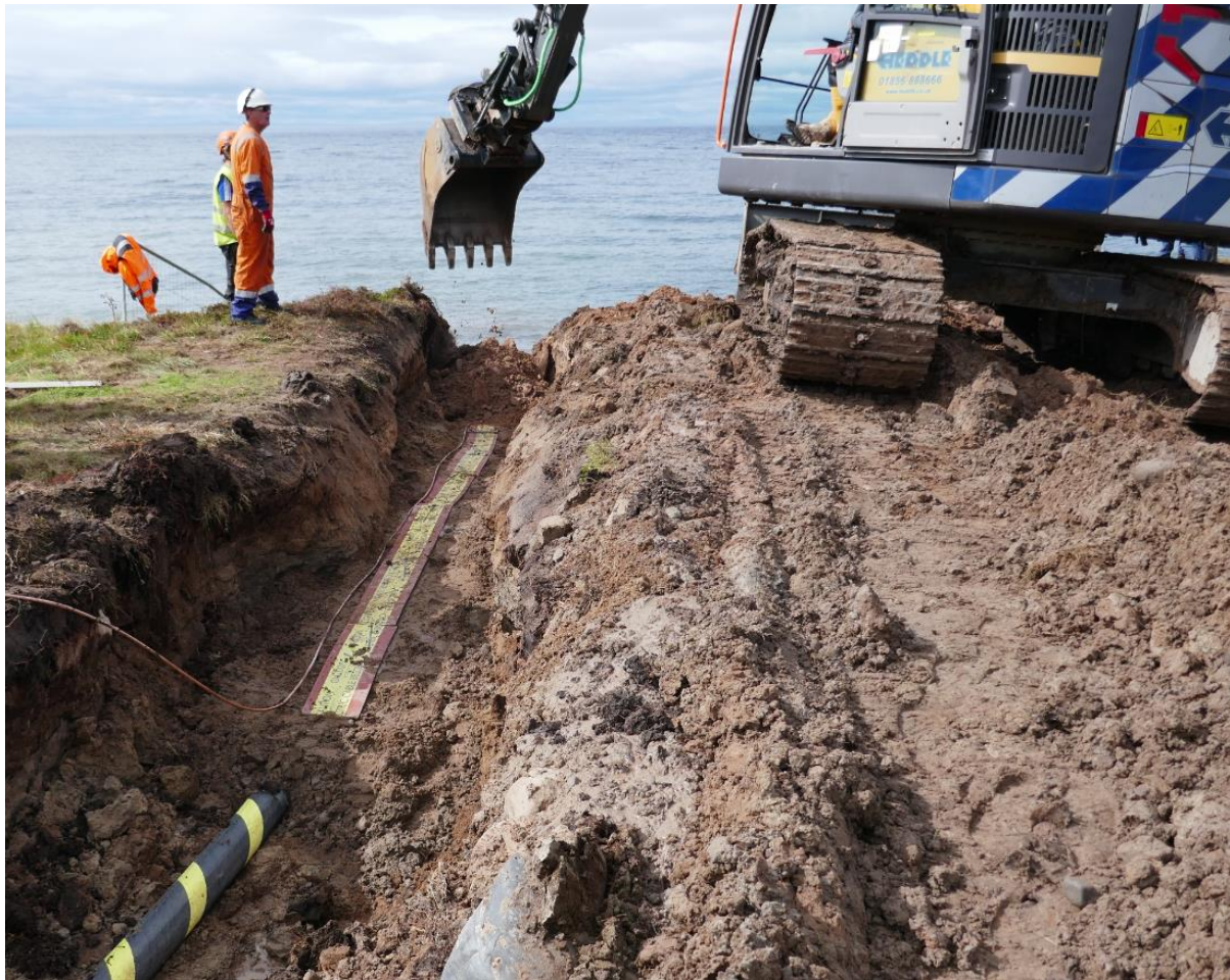
Figure 27: Bare Earth wire being installed in Subsea cable Trench
