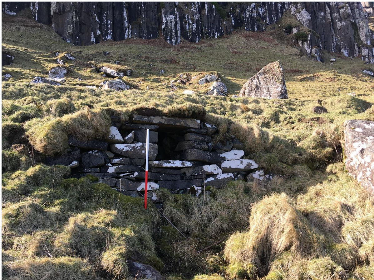
Figure 6.4.7: View west of drystone-built culvert (Site 57)
