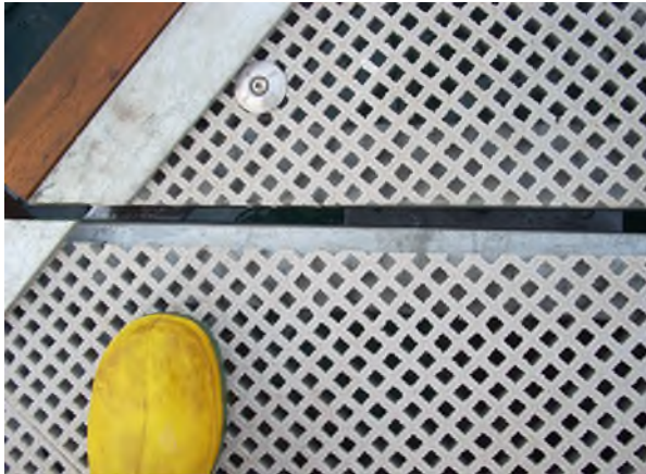
Figure 13.1.1: An Example of GRP Mini Mesh
