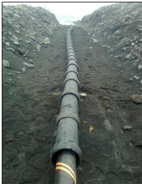
Figure 4-15 Example Split Pipe Installation
