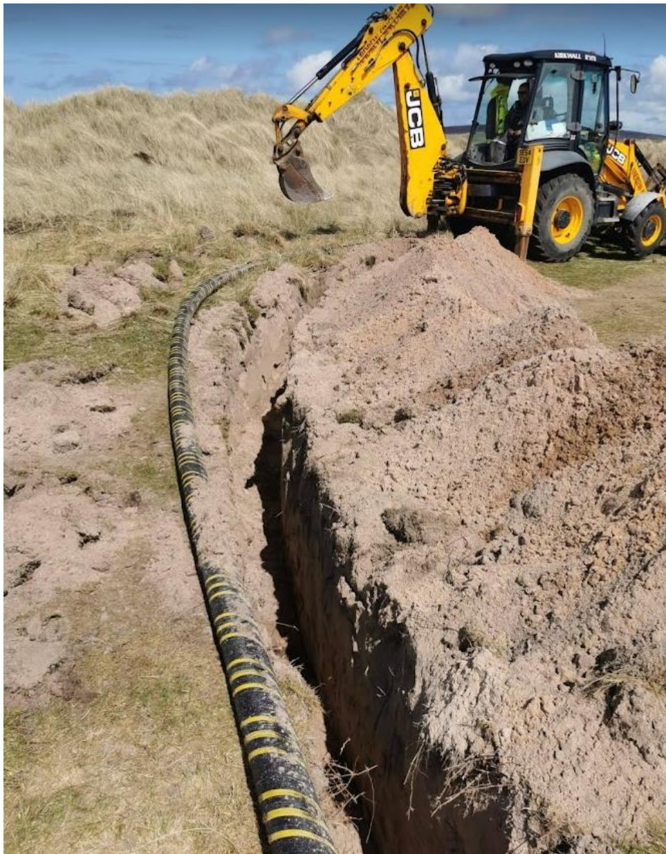
Figure 4-7 Example of OCT Cable Burial
