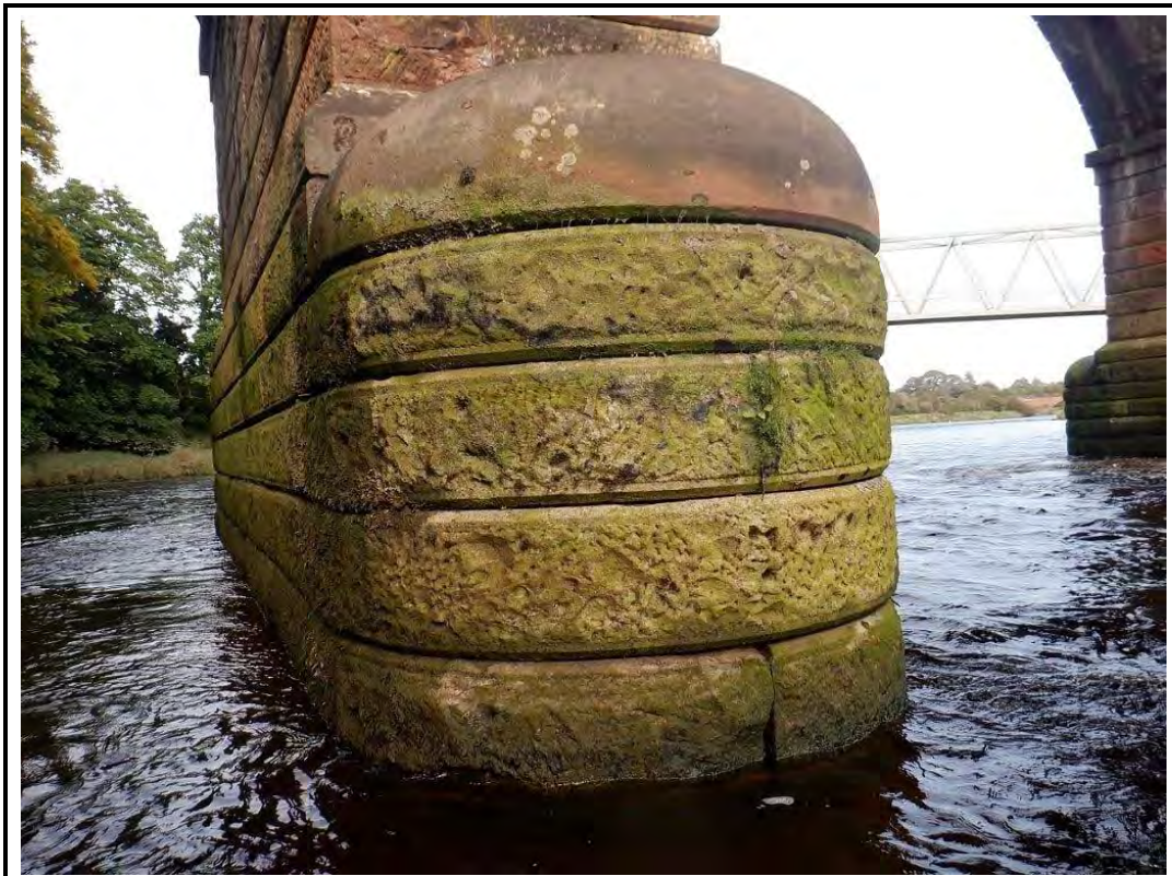
PHOTO 22: P22 - PIER 2 DOWNSTREAM NOSE 14/09/20
