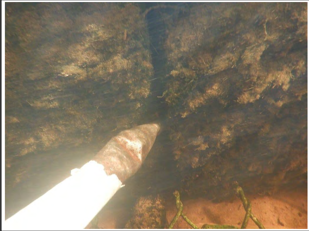
PHOTO 33: P33 - PIER 4 LM FACE 14/09/20
