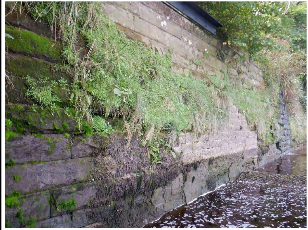
PHOTO 15: P15 - UPSTREAM LM RETAINING WALL 14/09/20
