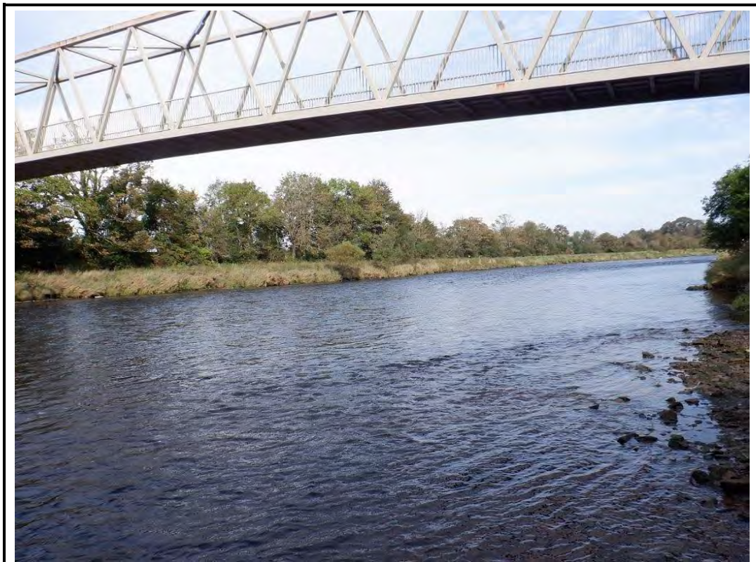
PHOTO 2: VIEW LOOKING UPSTREAM FROM STRUCTURE 14/09/20
