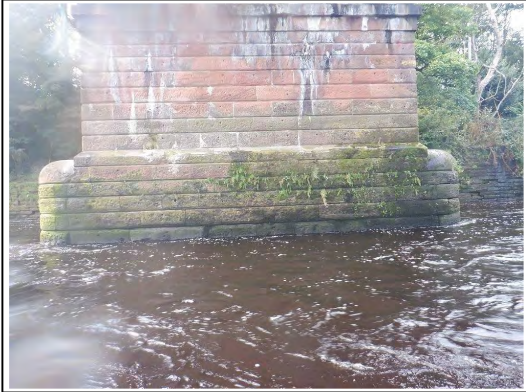
PHOTO 25: P25 - PIER 2 HM FACE 14/09/20
