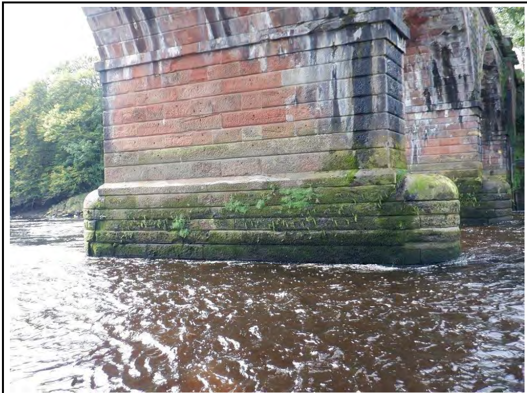
PHOTO 30: P30 - PIER 3 HM FACE 14/09/20
