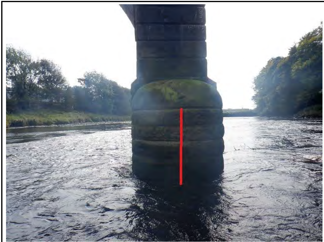
PHOTO 36: P36 - DATUM - PIER 3 UPSTREAM NOSE 14/09/20
