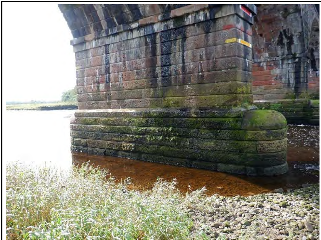
PHOTO 34: P34 - PIER 4 HM FACE 14/09/20
