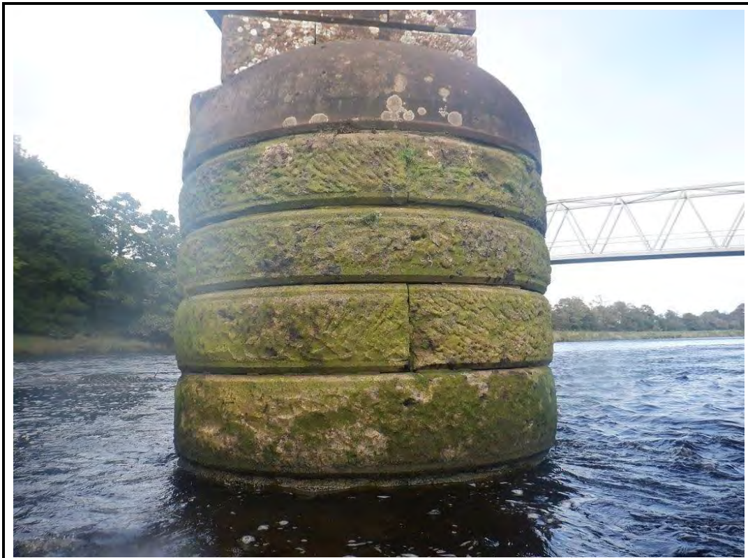
PHOTO 26: P26 - PIER 3 DOWNSTREAM NOSE 14/09/20
