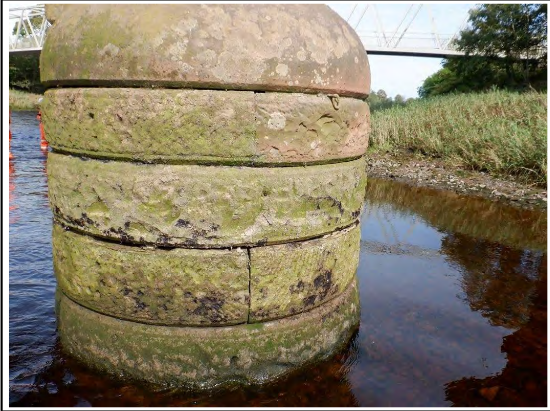
PHOTO 31: P31 - PIER 4 DOWNSTREAM NOSE 14/09/20
