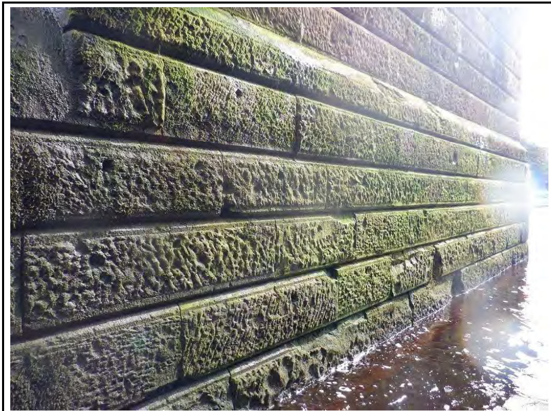
PHOTO 24: P24 - PIER 2 LM FACE 14/09/20
