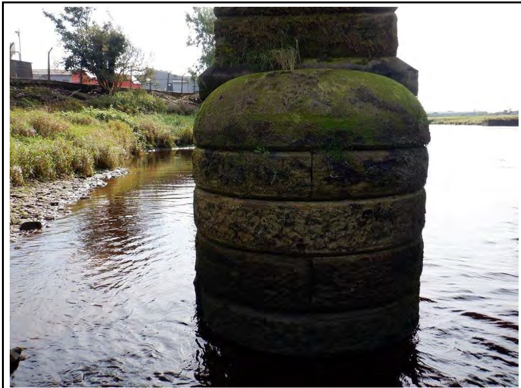
PHOTO 32: P32 - PIER 4 UPSTREAM NOSE 14/09/20
