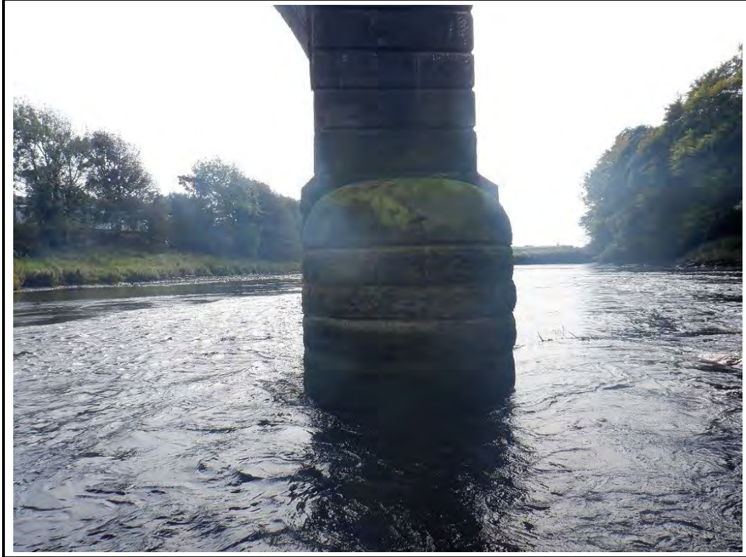
PHOTO 27: P27 - PIER 3 UPSTREAM NOSE 14/09/20
