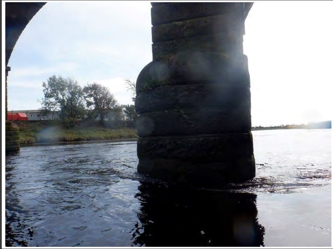
PHOTO 23: P23 - PIER 2 UPSTREAM NOSE 14/09/20
