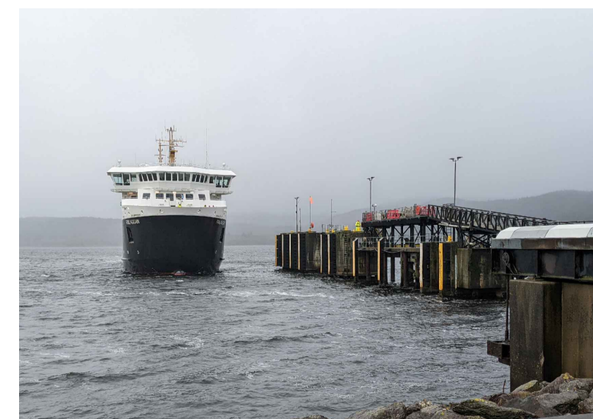
Image 9 General View of South Berth
