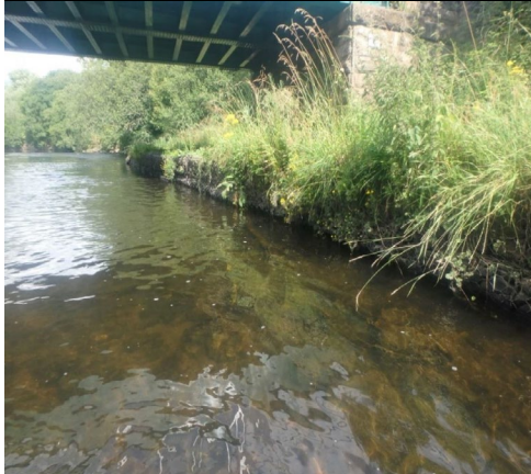
Key 2 - View of gabion retaining wall
