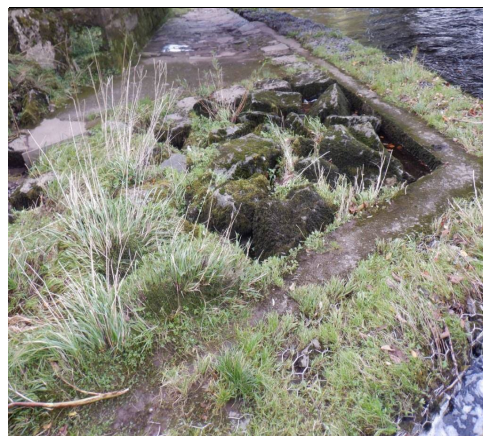
Key 7 -Location of work at upstream LM walkway
