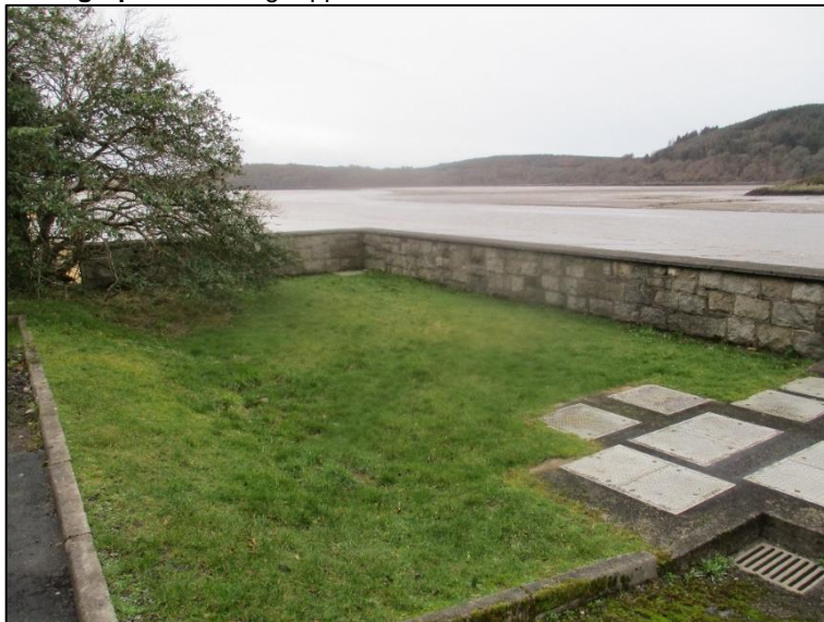
Photograph 1: Existing Kippford WwTW
