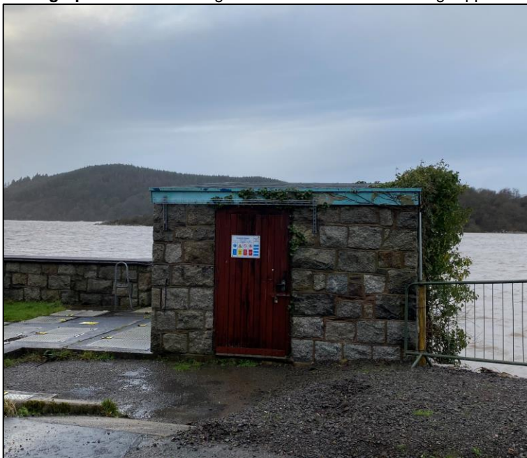
Photograph 5: Small building associated within the existing Kippford WwTW.
