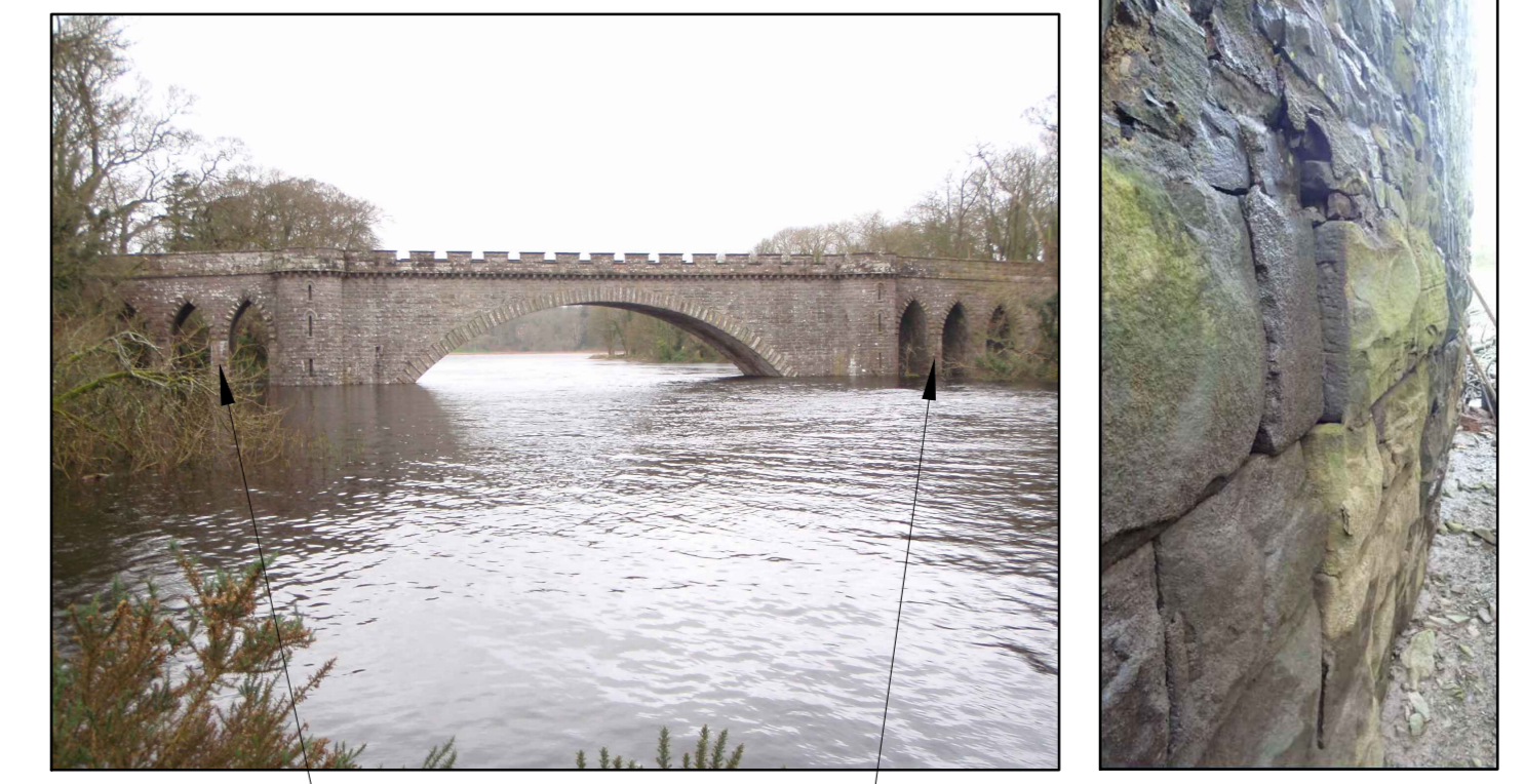
SIDE FACE (PART) SHOWING BULGING OF INTERMEDIATE PIER AT SOUTH END OF THE BRIDGE
