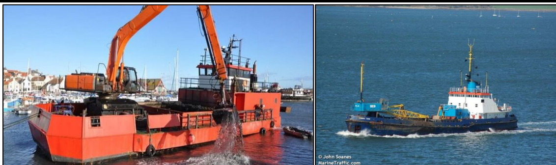
FIGURE 1.1 DREDGE VESSELS – WYRE SANDS AND CHERRY SAND
