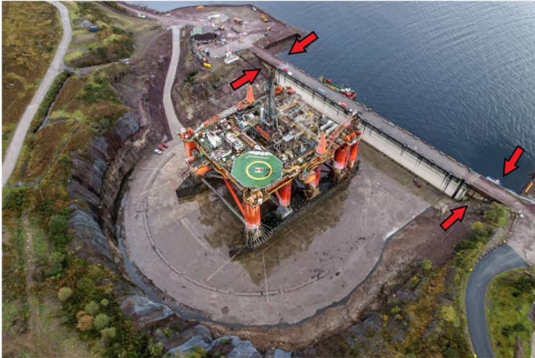
Figure 2.1: Dry Dock Abutment Locations (KPL, 2024)
