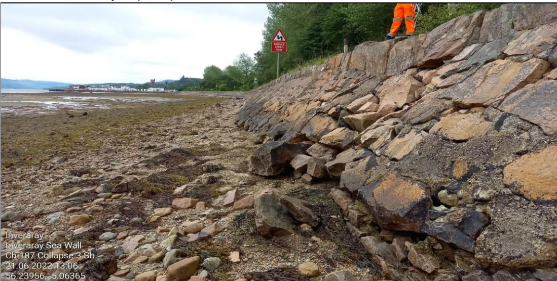
Ch.180 Wall collapse (No.3)
