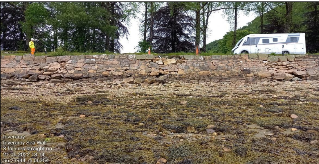
Ch.170 - Showing three localised areas where wall has collapsed
