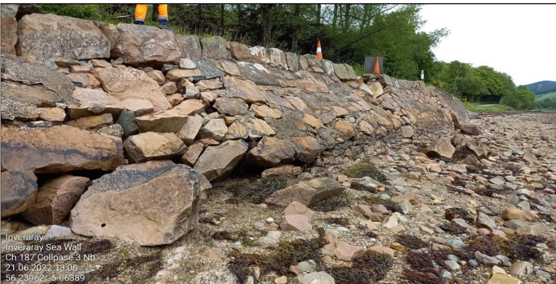
Ch.180 Wall collapse (No.3)
