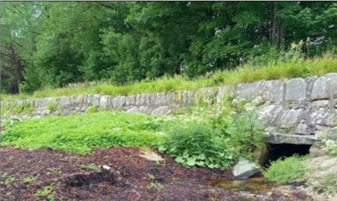
Ch.97 - Box culvert 1.1m L x 0.7m W
