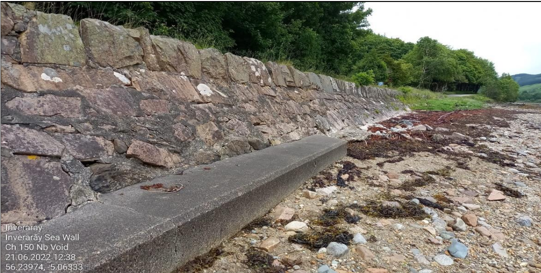
Ch.155 - End of concrete toe
