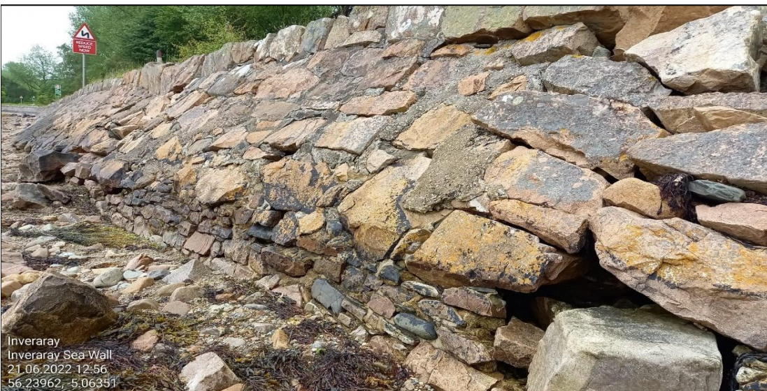
Ch.180 Wall collapse (No.2)
