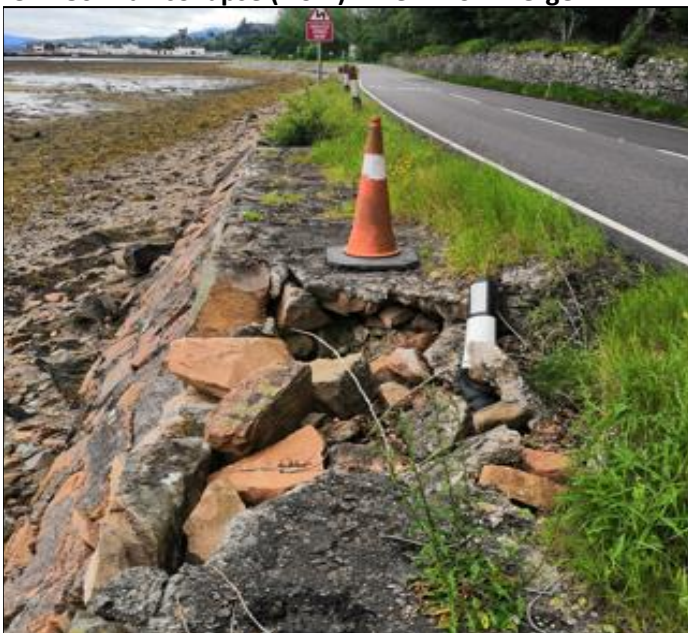
Ch.180 Wall collapse (No.2) - View from Verge
