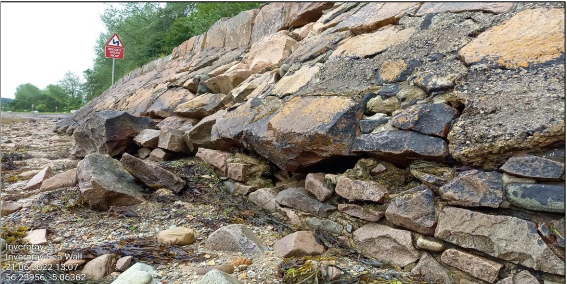
Ch.180 Wall collapse (No.3)
