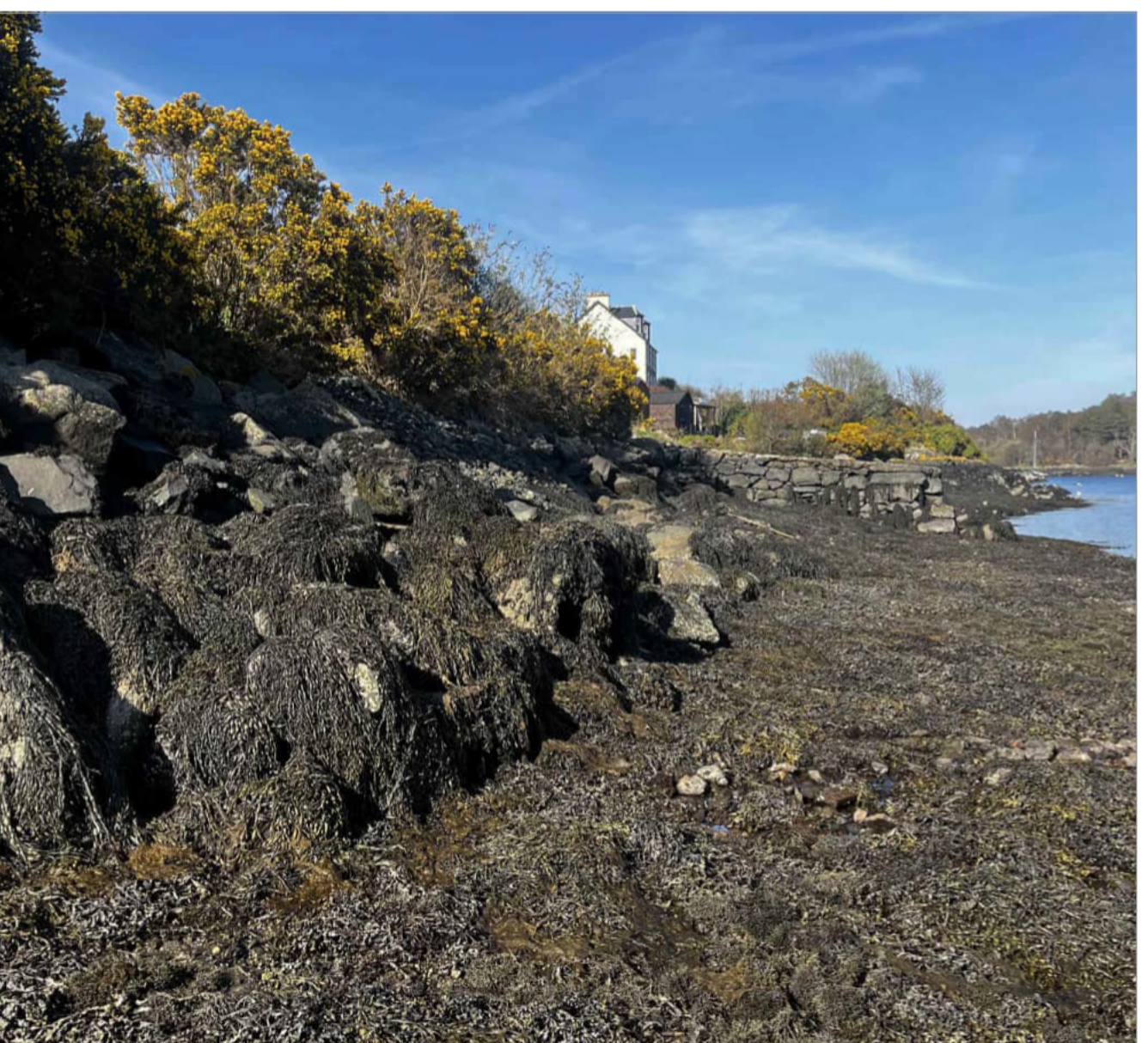
Photograph Nr.3 (11/04/2025): Revetment
