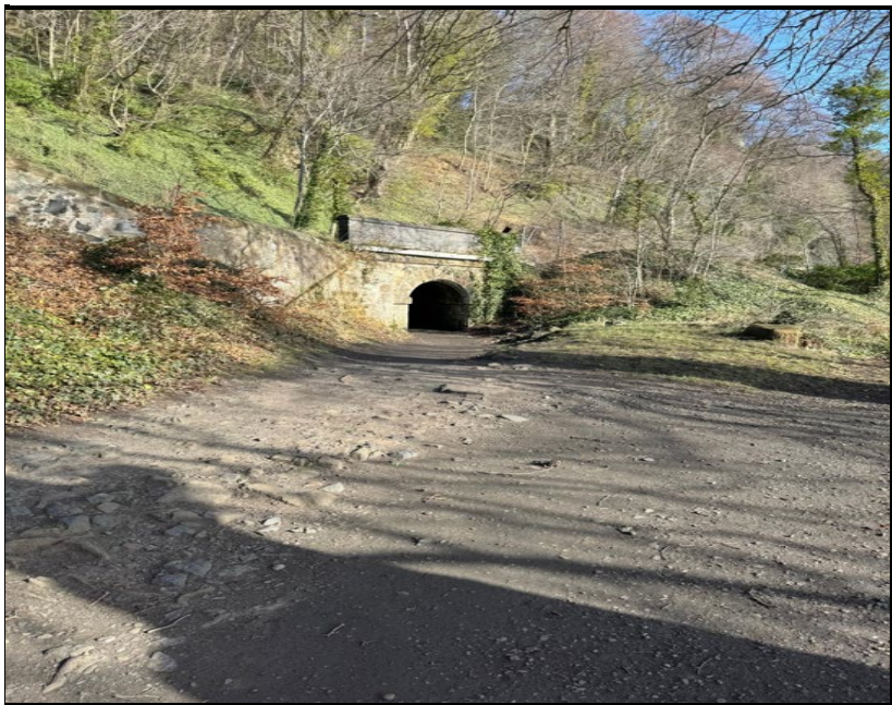
Key 4 - View of access path
