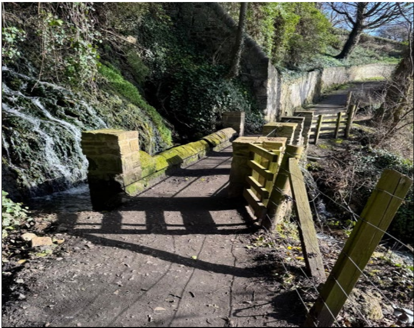
Key 5 - Vie of bridge on access path
