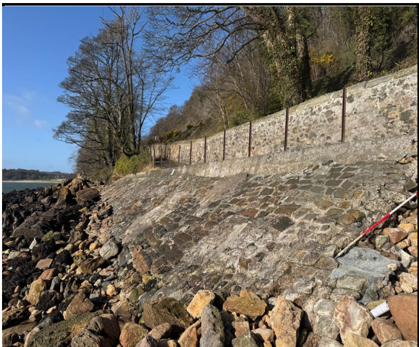
Key 2 - View looking from the scour
