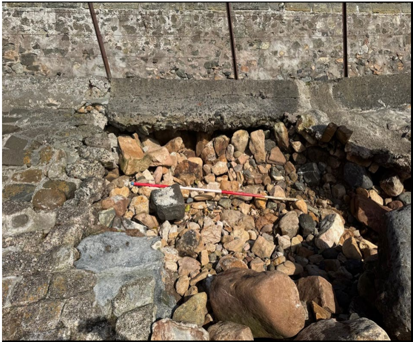
Key 1 -Scour 3m with x 3m length x 600mm depth
