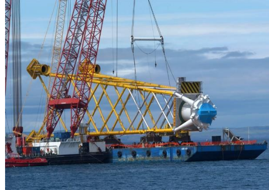
Figure 5.9 – Example of a jacket substructure being transported in horizontal position on a transportation cargo barge and lifting from cargo barge
