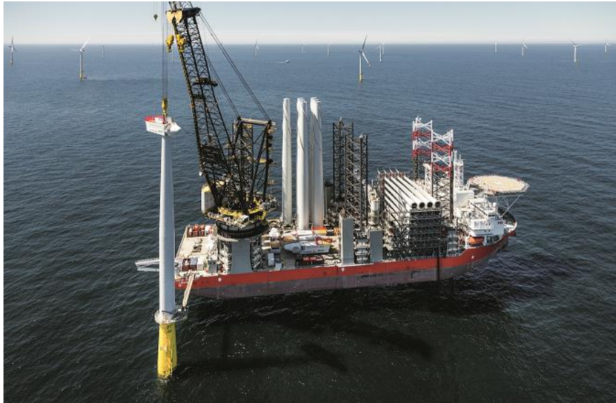
Figures 5.22 - A typical nacelle lifting and installation process
