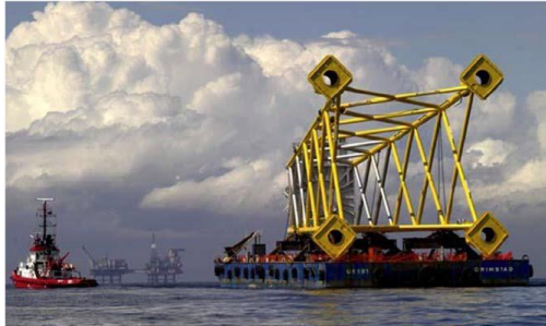
Figure 5.9 – Example of a jacket substructure being transported in horizontal position on a transportation cargo barge and lifting from cargo barge
