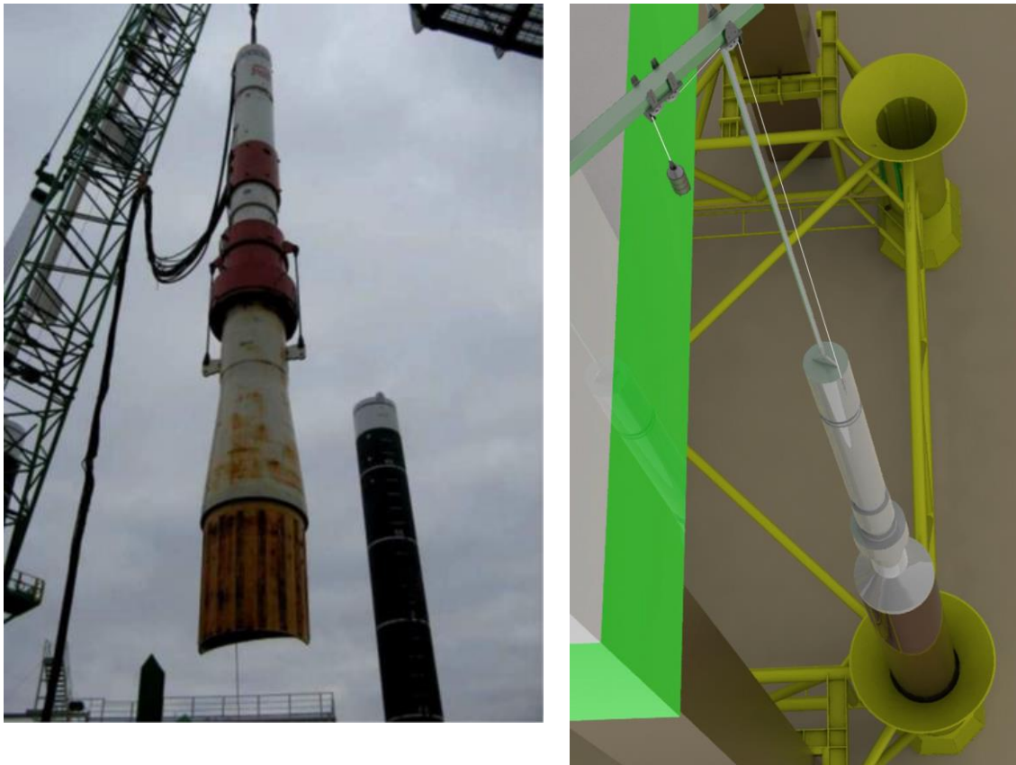
Figure 5.7 – Example of a piling hammer (with follower) and subsea hammer on pile and piling through the PIF
