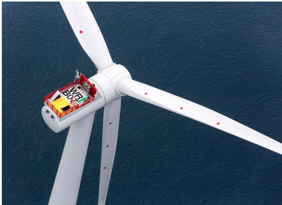
Figure 6.1 – Example of blade hover marks installed at the Westernmost Rough Offshore Wind Farm
