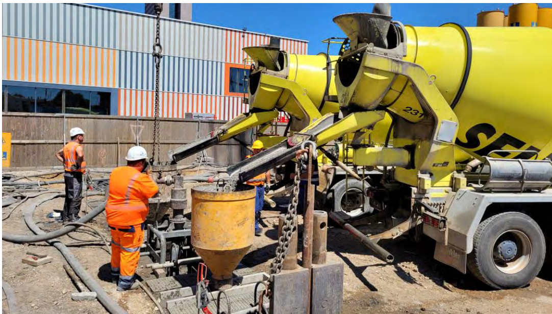
Figure 17: Tremie pipe & hopper assembly in trap over panel
