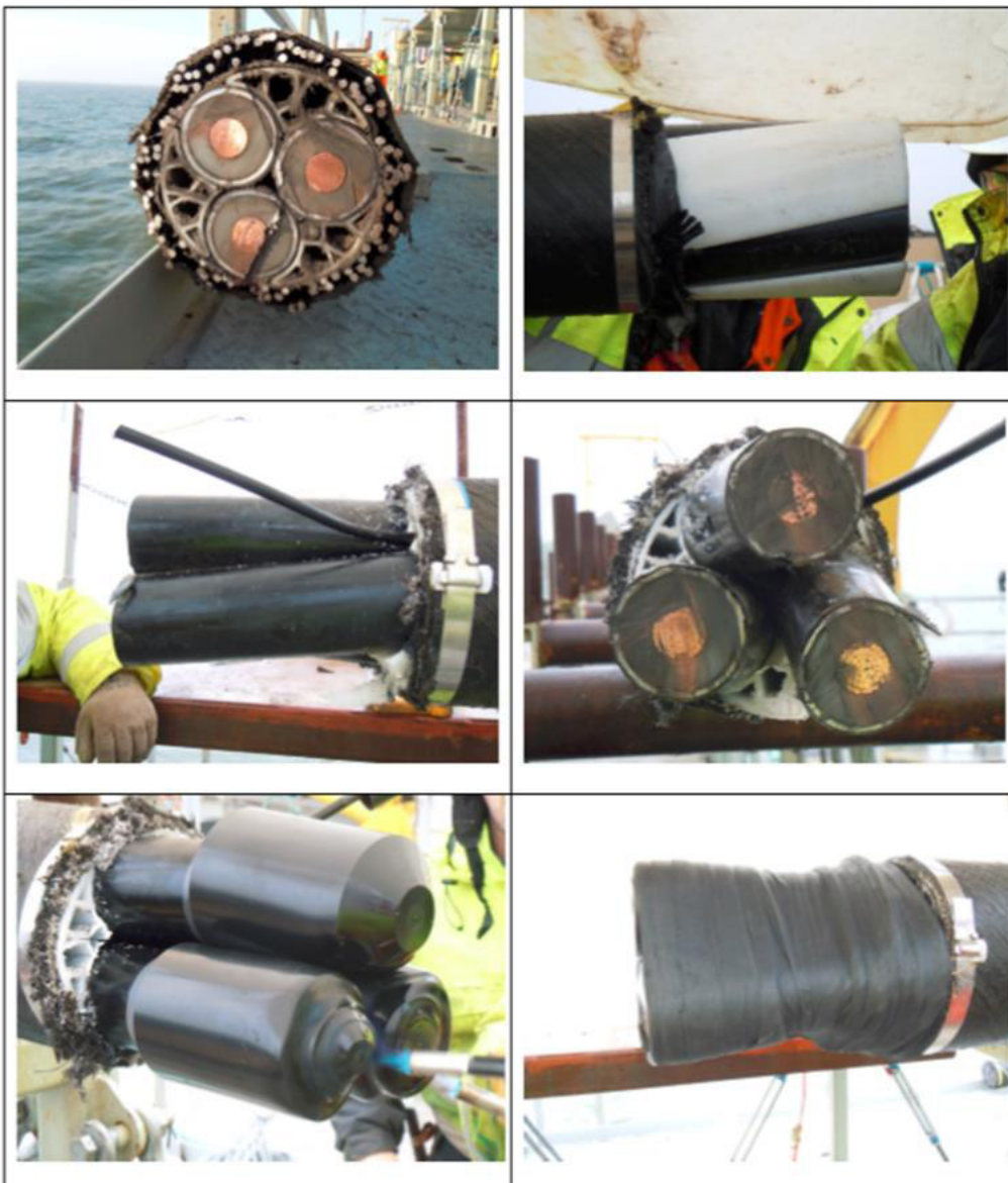
Figure 9.5 - Typical cable cutting and sealing process
