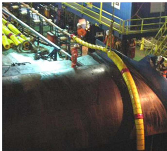
Figure 9.4 - Example of a cable laying operation (cables first end being over-boarded from the cable laying vessel)
