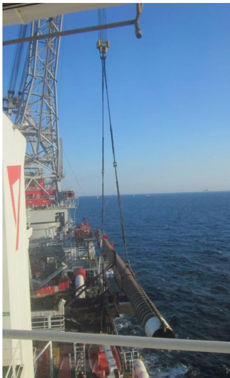
Figure 5.7 – Pile being up-ended ready for deployment and being deployed into the PIF
