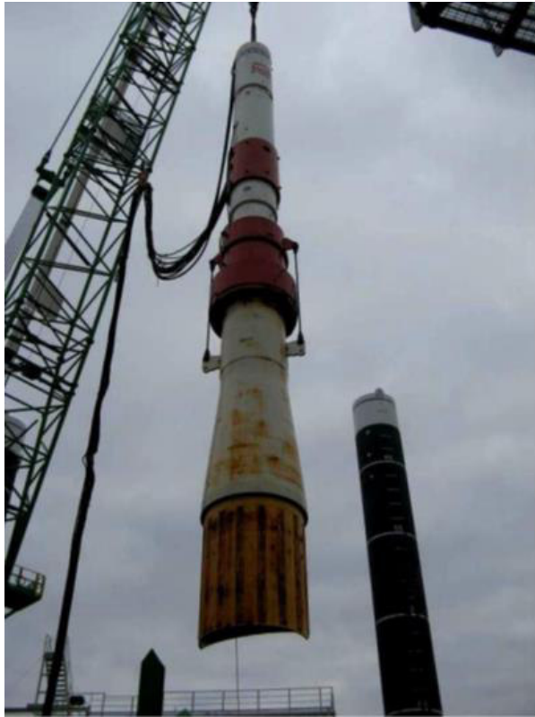
Figure 5.8 – Example of a piling hammer (with follower) and subsea hammer on pile and piling through the PIF
