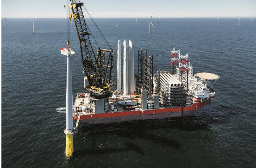
Figures 5.24 - A typical nacelle lifting and installation process
