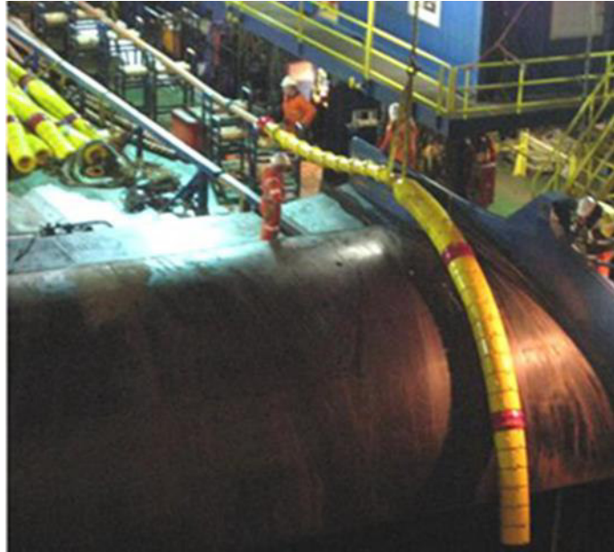
Figure 5.15 - Example of a cable laying operation (cables first end being over-boarded from the cable laying vessel)
