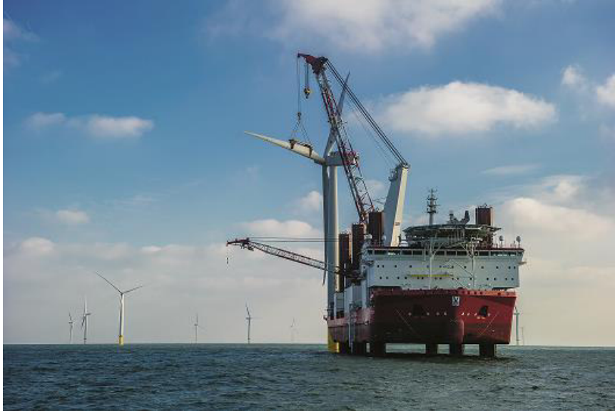
Figures 5.25 - A typical blade installation process
