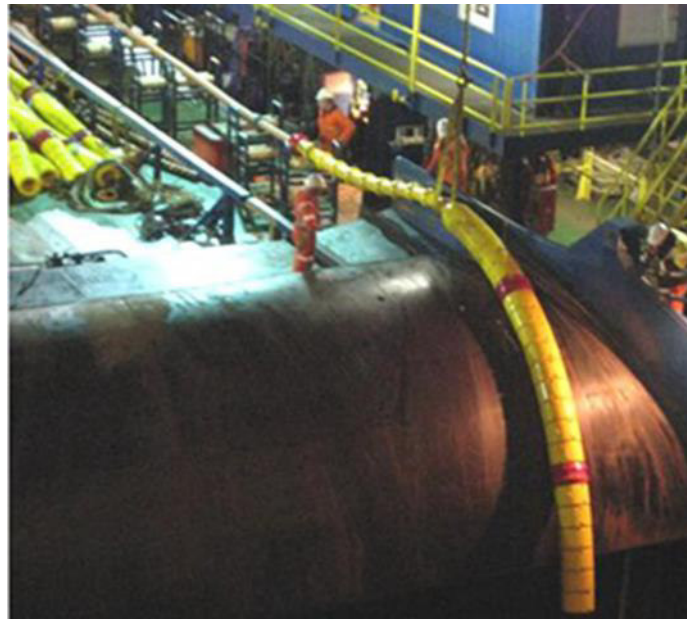
Figure 9.6. Example of a cable laying operation (cables first end being over-boarded from the CLV)
