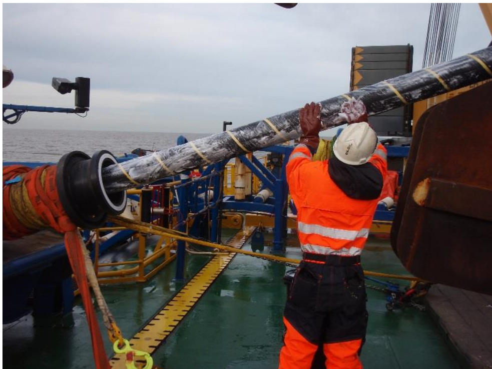
Figure 13 Example of a cable pull in into a HDPE duct end
