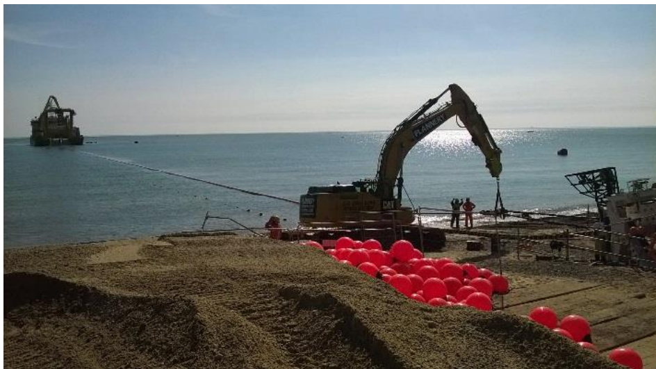
Figure 20 Example of a cable float in
