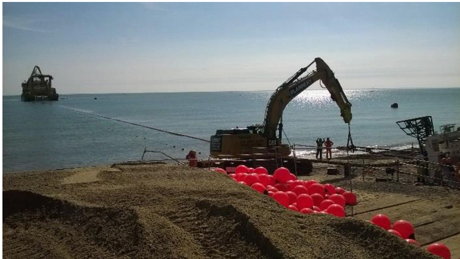
Figure 15 Example of a cable float in
