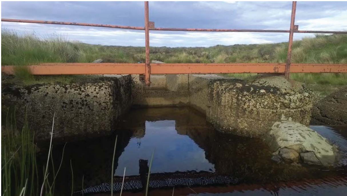
Figure 2: Impassable Weir (River Creed Catchment) at Loch an Ois (Downstream View)
