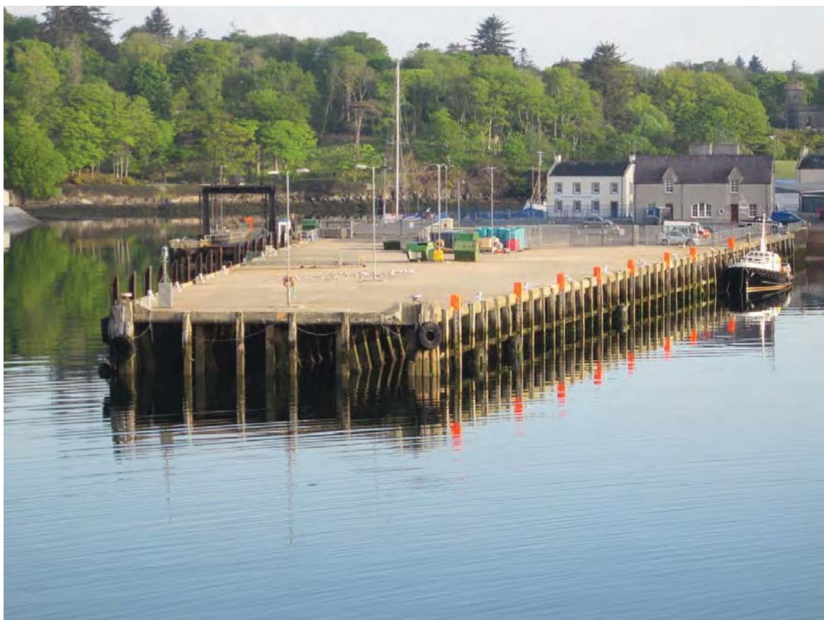
Figure 2.3: Open piled section of the outer part of No 1 pier
