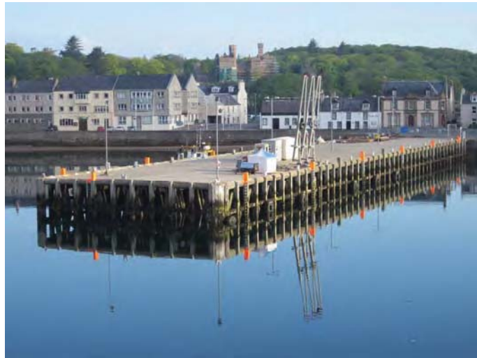
Figure 2.4: Open piled structure of the pier at South Beach (No 2 pier)
