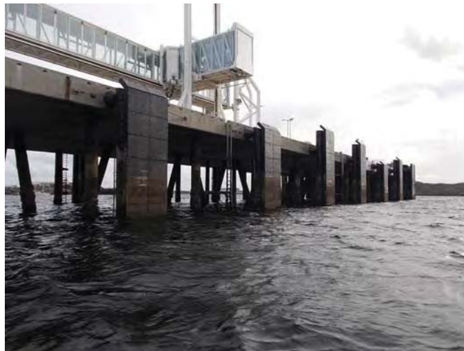
Figure 2.5: Tubular steel piled structure supporting the Stornoway Ferry terminal pier
