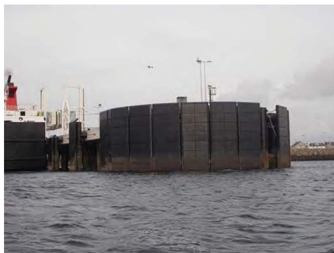
Figure 2.6: Semi-circular fender wall at the end of the ferry terminal pier
