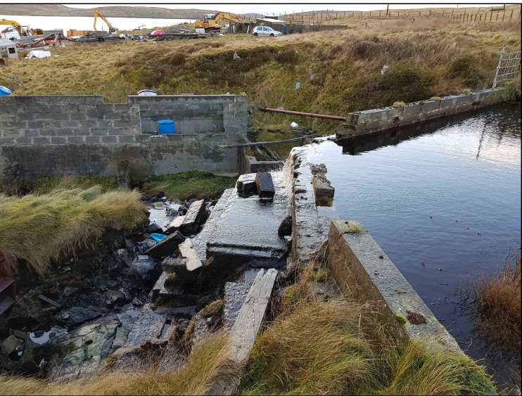
EXISTING CONCRETE DAM TO BE REPAIRED WITH WORKS INCLUDING HEIGHTENING DAM BY APPROXIMATELY 400mm (PROPOSED OVERFLOW LEVEL +7.85 ACD). DAM TO BE EXCAVATED
