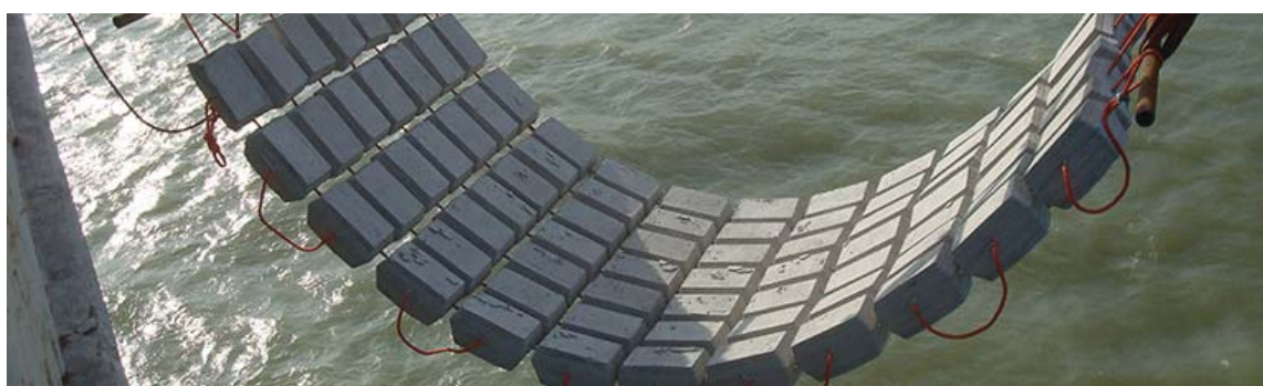
Figure 2-3 Concrete mattress
