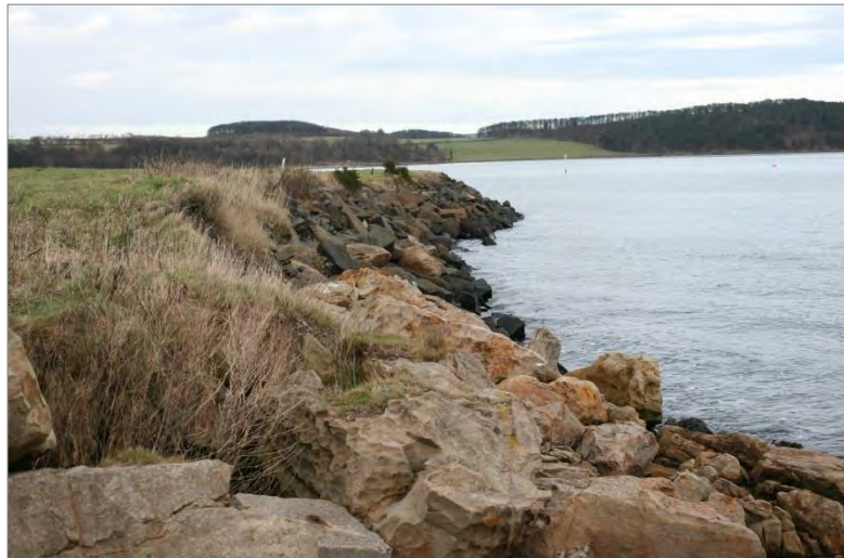
Image 2-1 Headland: Existing Rock Armour
