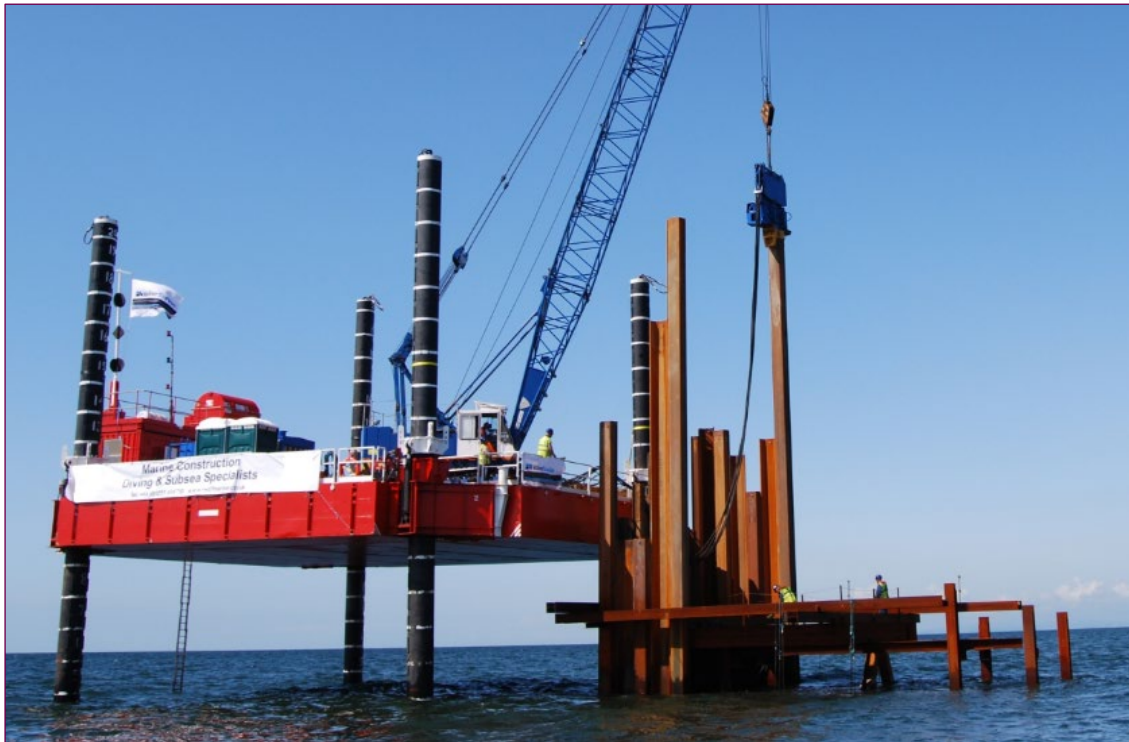
Figure 2.6: Typical Jack-Up Barge Completing Marine Piling
