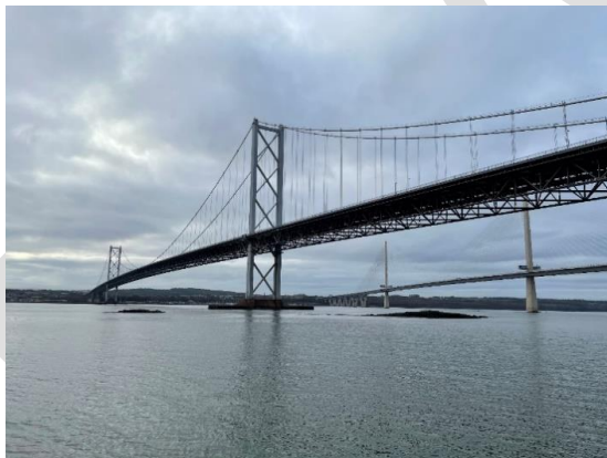
Photograph 1: View of the Forth Road Bridge from the north east looking towards South Queensferry, with the Queensferry Crossing visible in the background.
