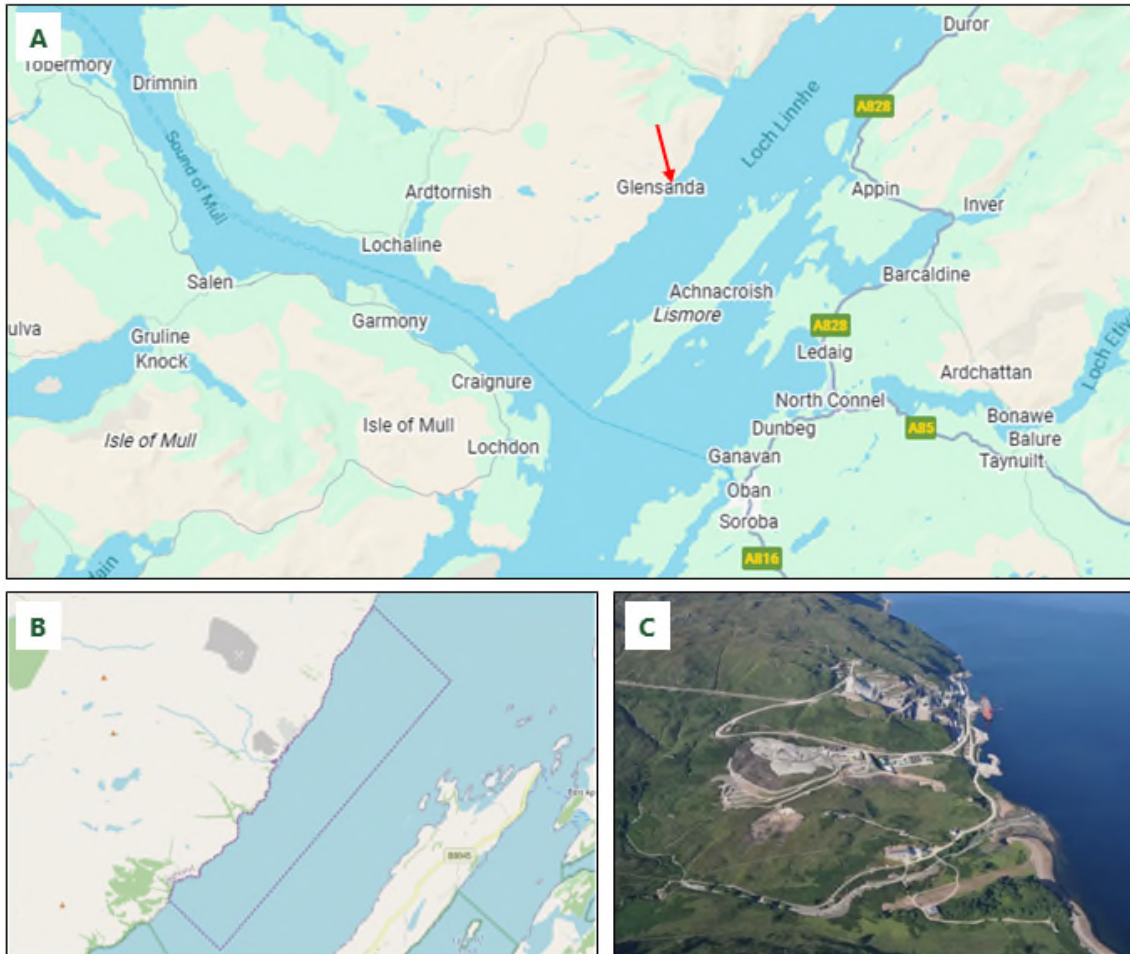
Figure 2.1.1: (A) Location of the Port of Glensanda (red arrow), (B) statutory limits of the Port of Glensanda (purple dashed line), (C) aerial view of the Port (Holcim UK, 2025a)
