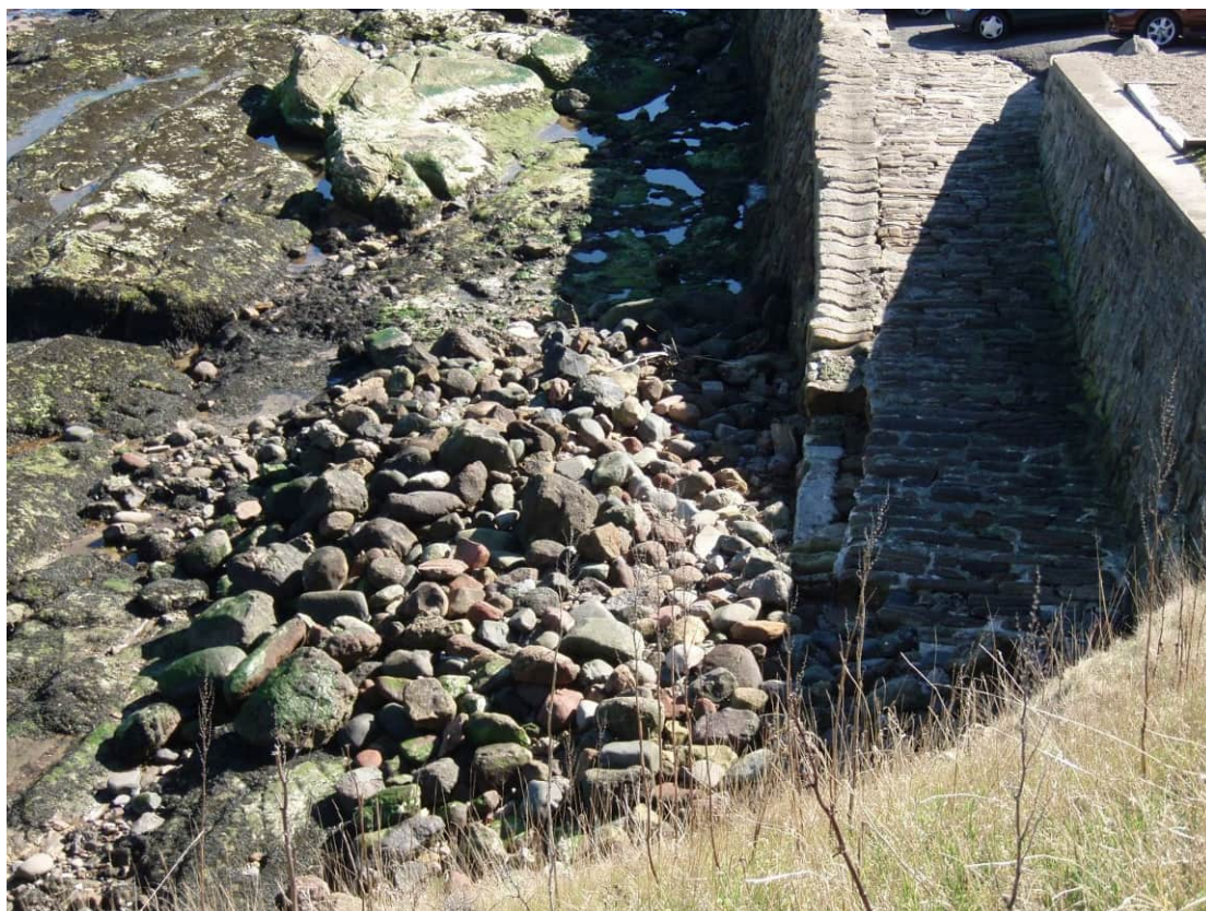
Boulders moved by the sea and up against the side and base of the slipway. March 2007.
