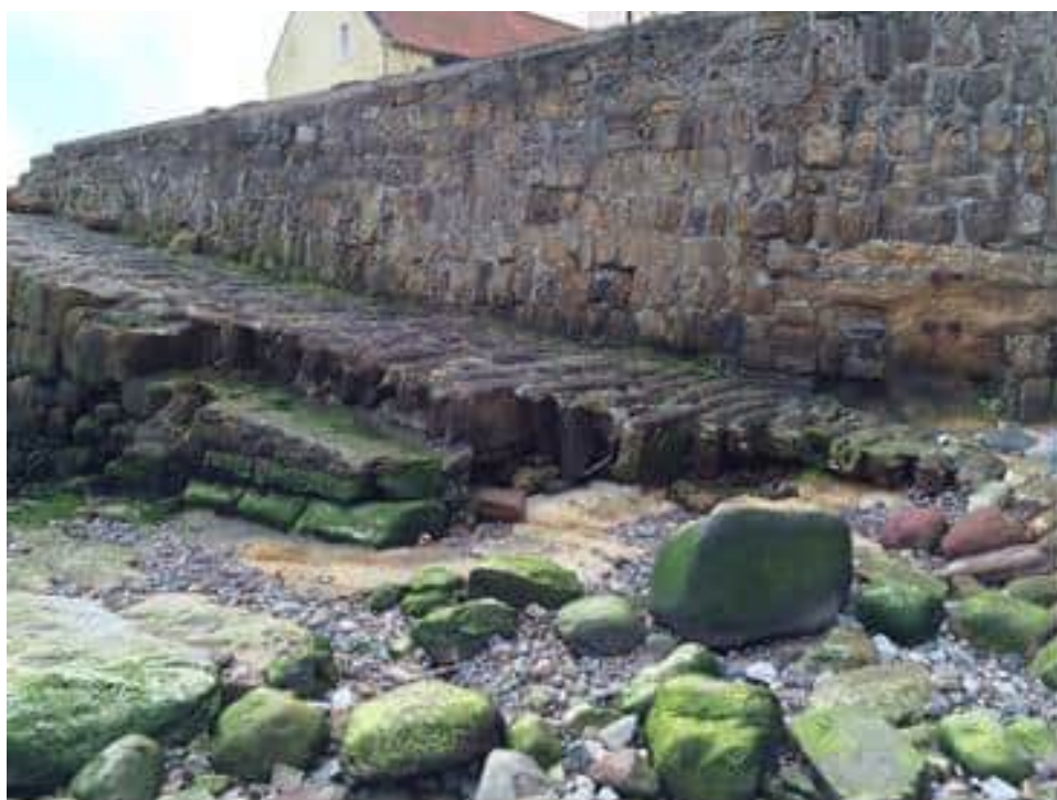
Sea action is starting to break away at the lower section of the slipway. March 2015.
