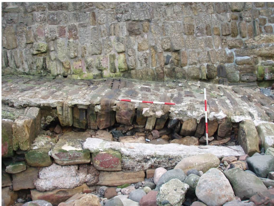
Damage to the surface of slipway by mobile boulders. March 2007.
