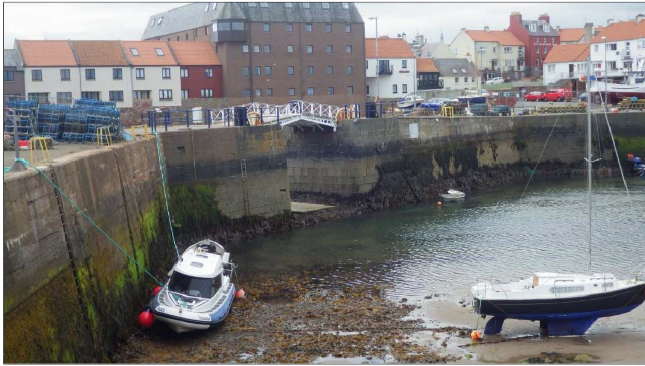
PHOTO OF EXISTING SLIPWAY RAMP LOOKING SOUTH
