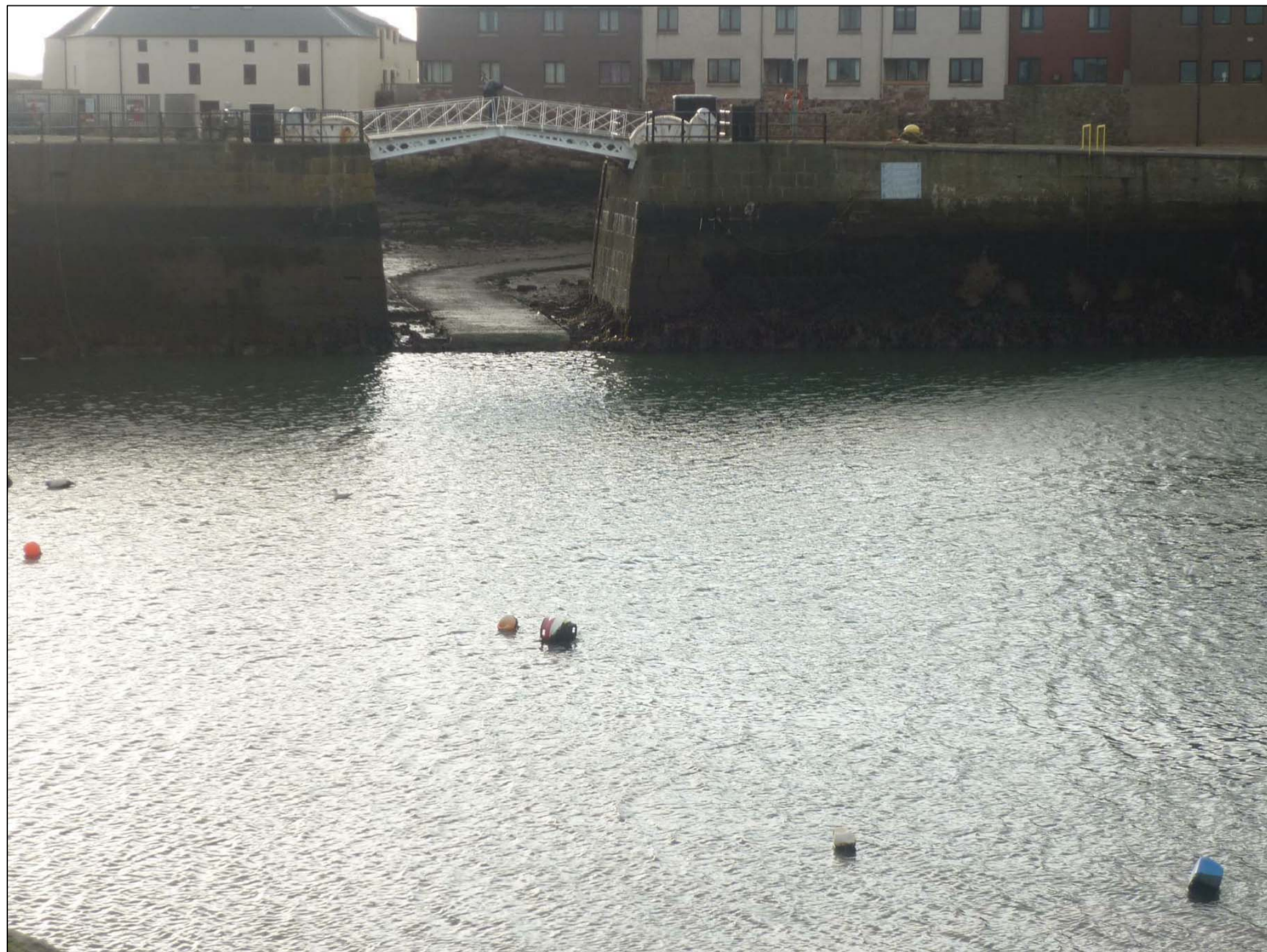
PHOTO OF EXISTING SLIPWAY RAMP LOOKING EAST
