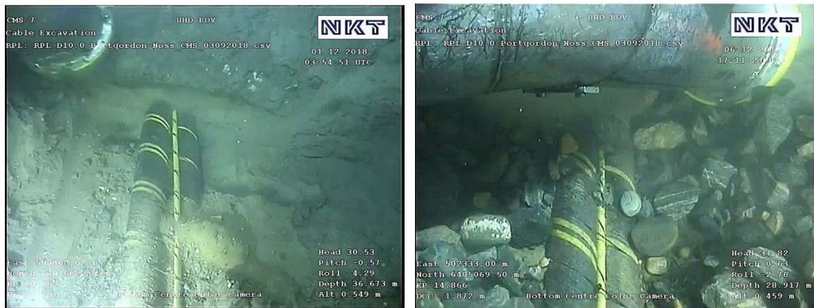
Figure 3-2 Cable Excavation and Inspection KP 10.929 (left), KP 14.866 (right)
