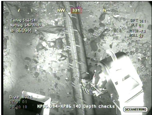
Figure 3-3 Cable Excavation and Inspection, KP 86.
