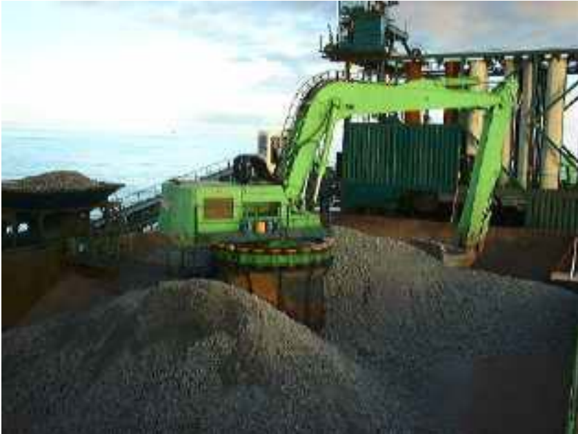
Figure 5-2 Excavator onboard the vessel
