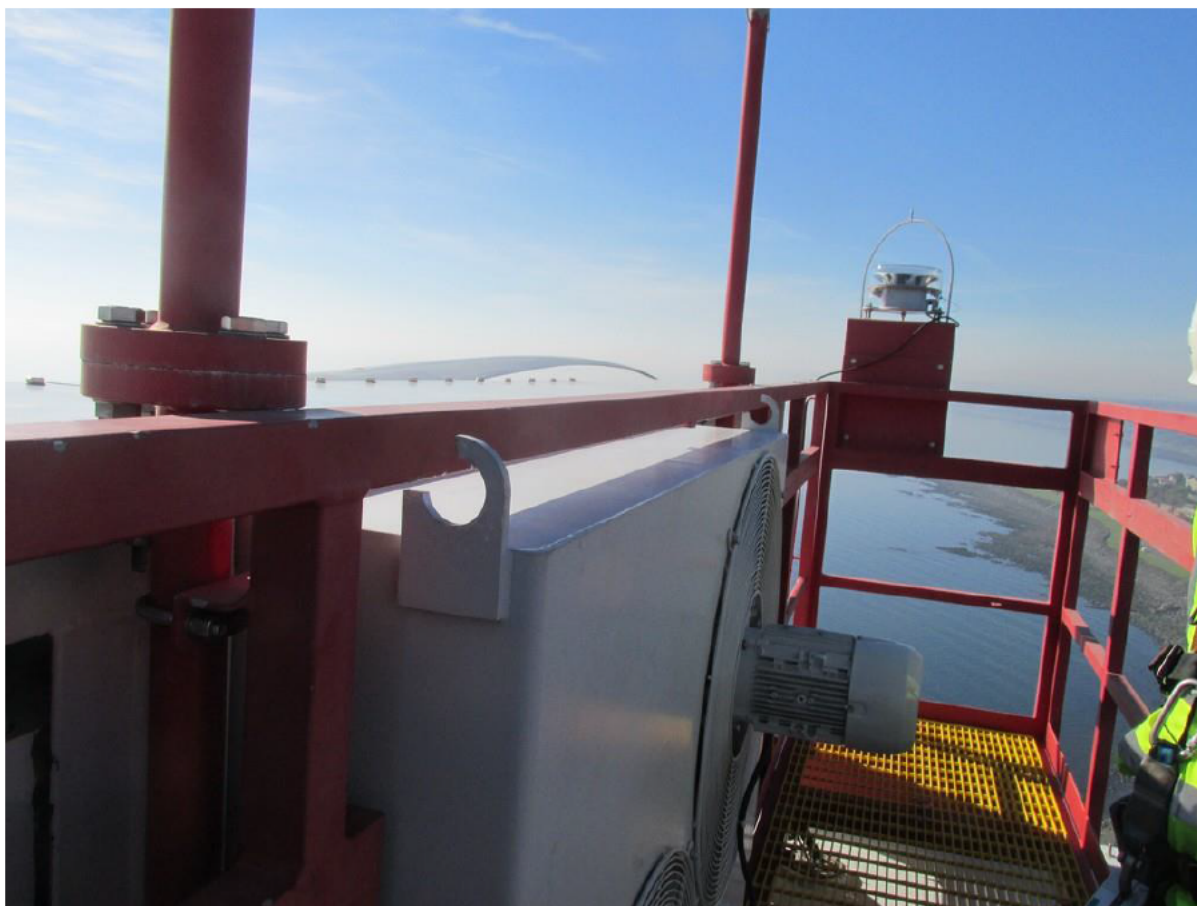
Figure 6-6: WTG Roof Enclosure with Aviation Light
