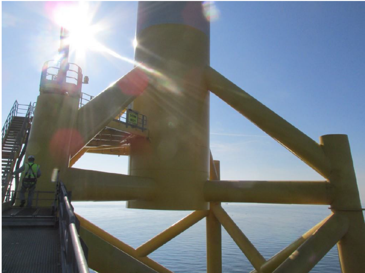
Figure 6-9: WTG Transition Piece and Access
