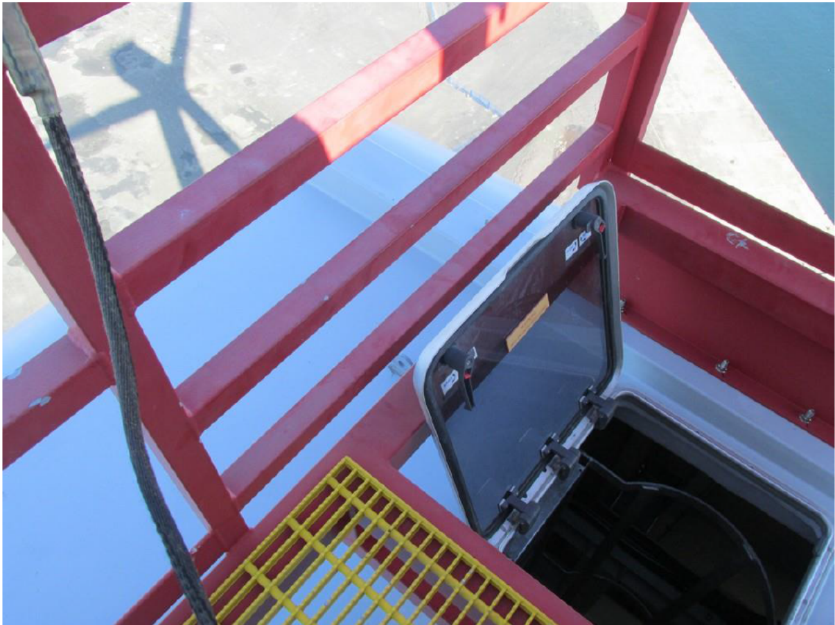
Figure 6-7: WTG Roof Enclosure Access Down to Nacelle
