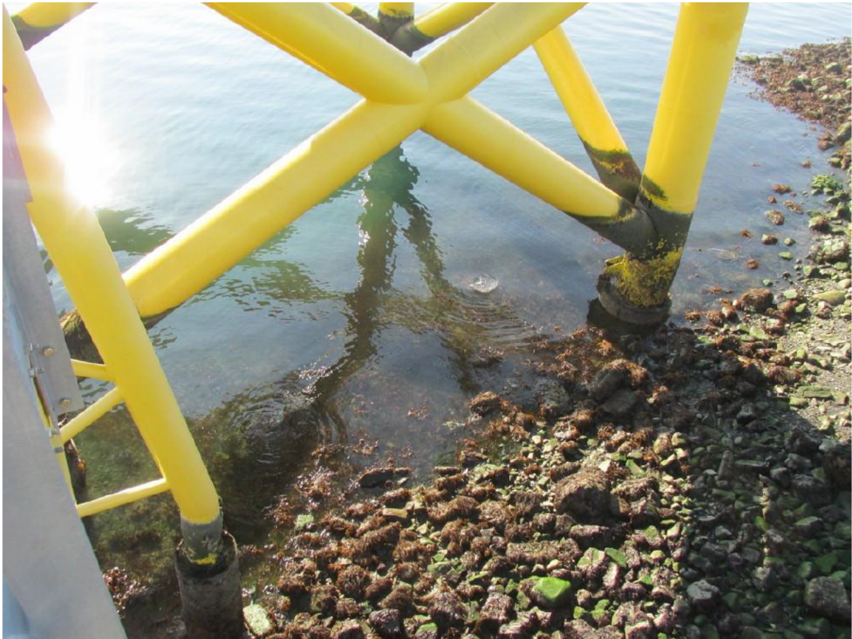
Figure 6-8: WTG Foundations at LAT
