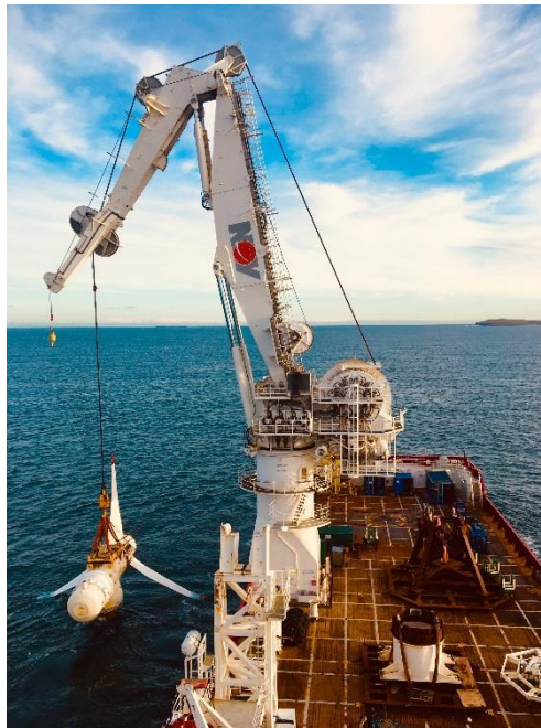
Figure 3 AR1500 in suspended from a 250Te AHC crane aboard the Seabed Stingray awaiting slack tide for installation.
