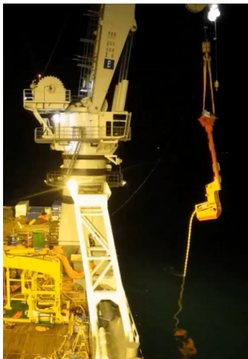
Figure 4 Lower CMS with export cable attached during installation
