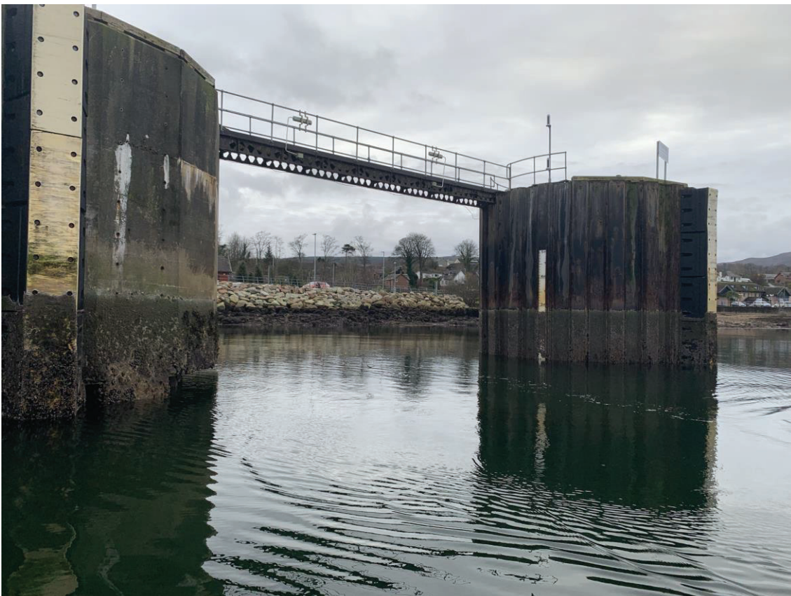
Figure 3 Inner mooring dolphin (left) and outer berthing/mooring dolphin (right) from north
