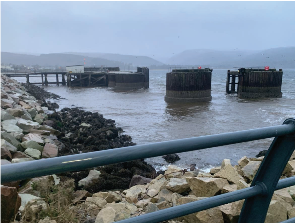
Figure 10 Pier head, inner lifting dolphin (left) and outer lifting dolphin (right)
