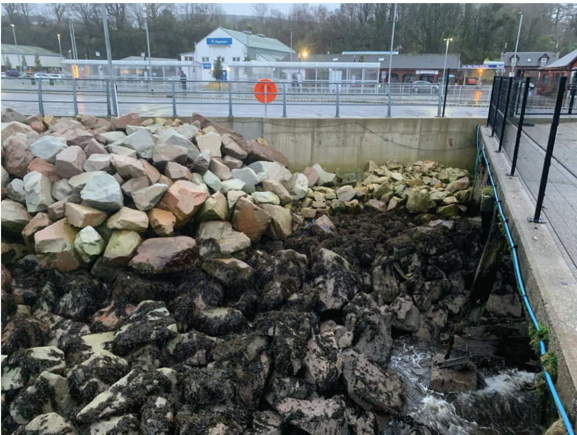
Figure 9 Pier approach to marshalling area from pier head, showing revetment to be completed
