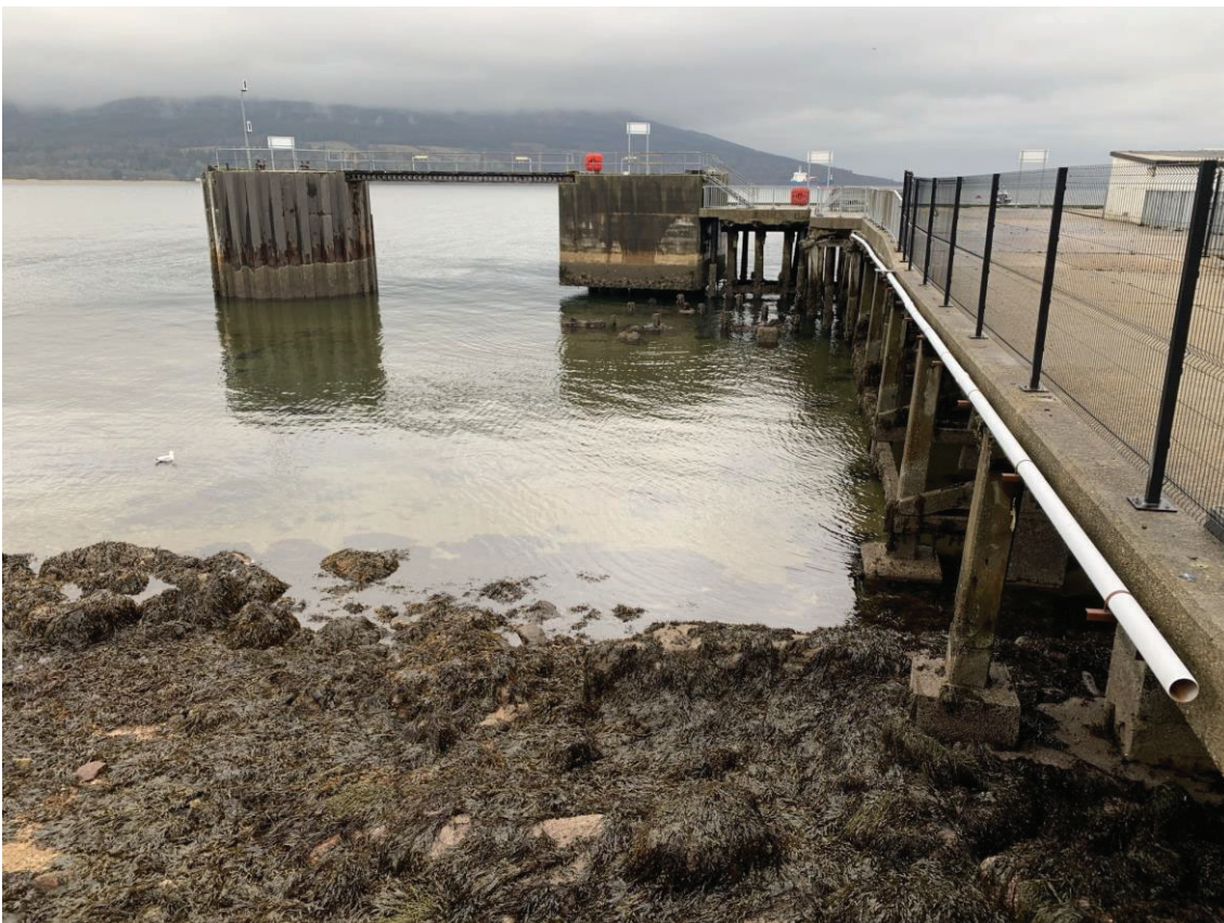
Figure 5 West side of pier approach and berthing/mooring dolphins from marshalling area
