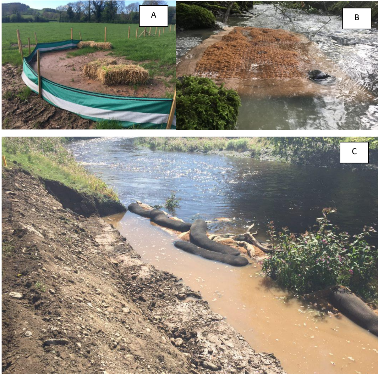
Figure 2. Examples of silt fence (A), silt mat (B) and silt wattle (C). Photo courtesy of Hy-Tex (UK) Limited and Salix Ltd.
