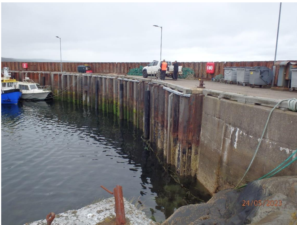
Photo 2 – View of existing quayside at proposed pontoon access bridge location
