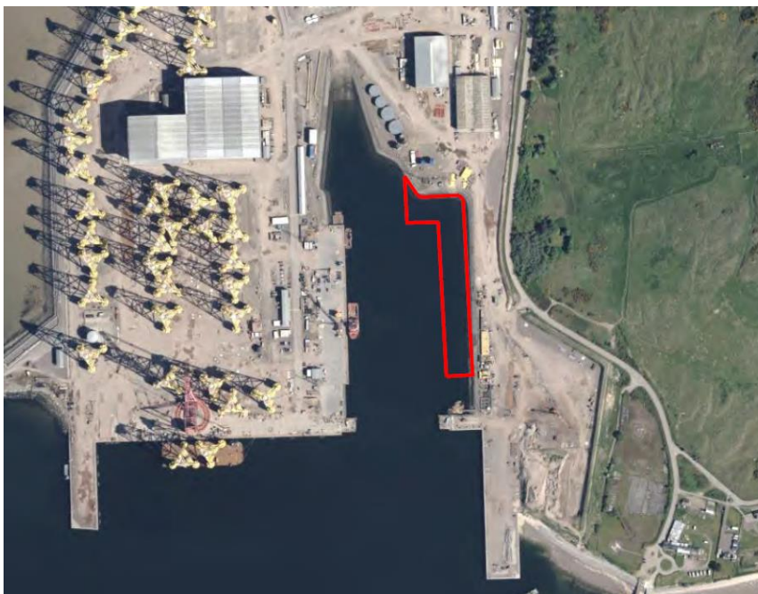
Plate 7-1: Aerial View of Nigg Energy Park showing the footprint of the temporary working platform
