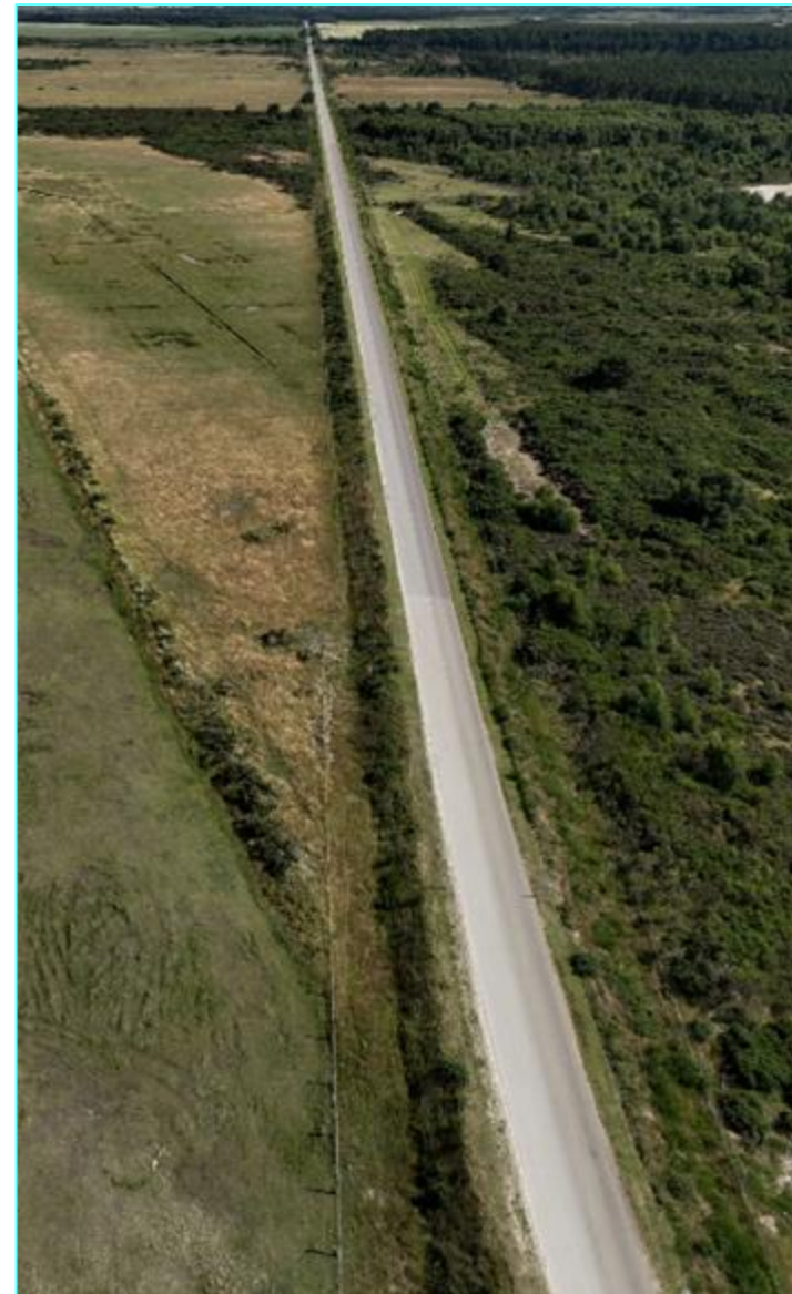
Left: Aerial photo of access road between security buildings
