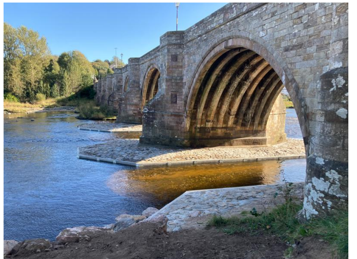
Showing completed scour protection including stone pitching to aprons 2025 season information 2025 season
