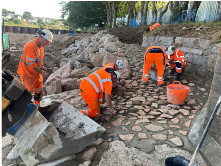
Showing completed scour protection including stone pitching to aprons 2025 season information 2025 season
