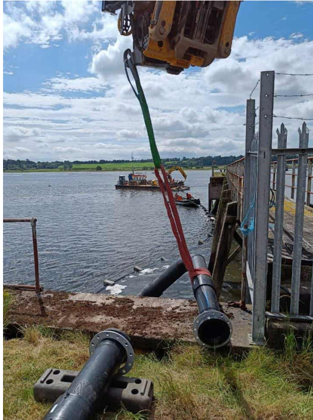
Figure 3 – Installation of the Temporary Discharge Pipe at Bowling (June 2022)
