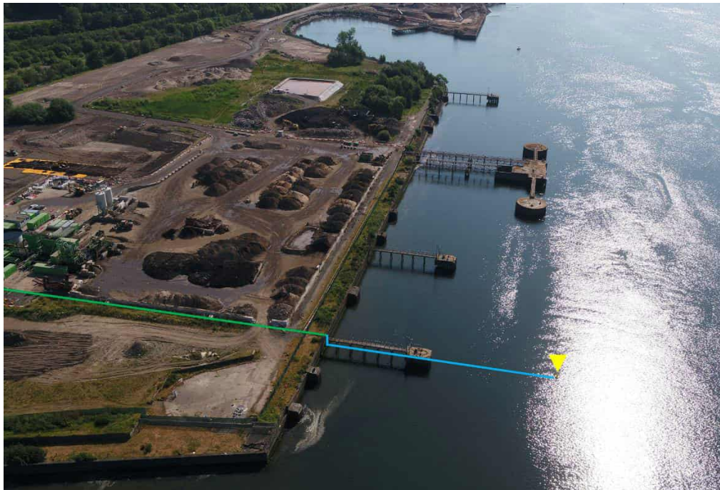
Figure 4 Temporary Discharge Pipe location - onshore section (green line), offshore section (blue line) and marker buoy (highlighted in yellow)
