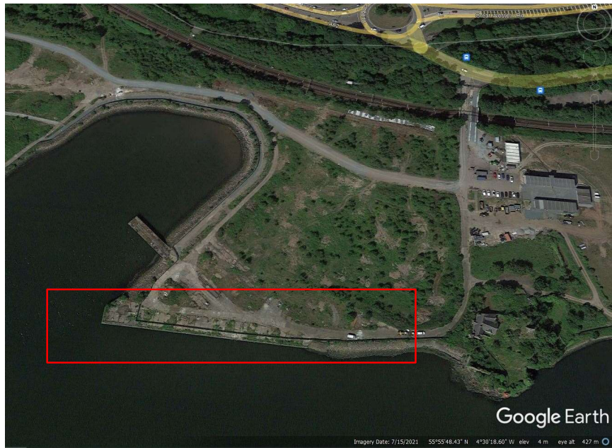
Figure 2 – Location of the existing coastal defence
