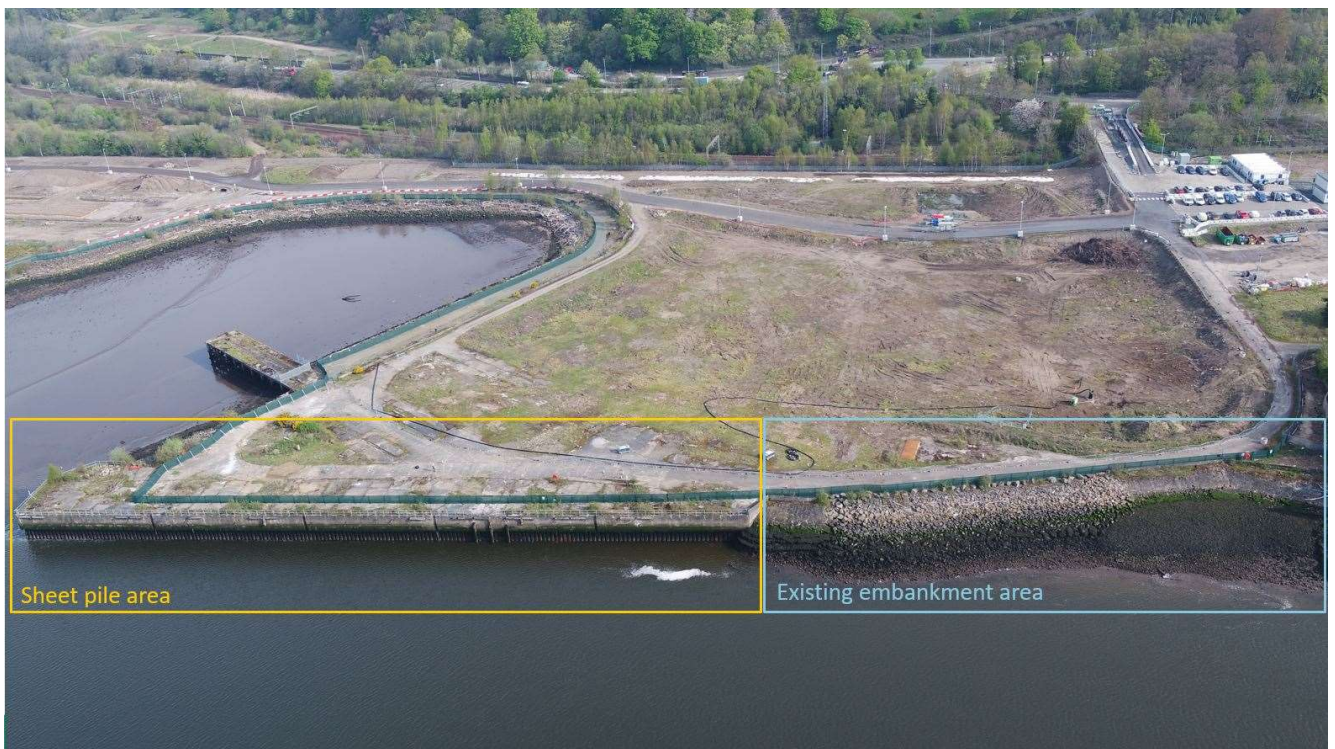
Picture 1 – Aerial view of the existing revetment structures with highlight of the sheet piles area (orange) and rock armour section (embankment area & OBB) (blue)
