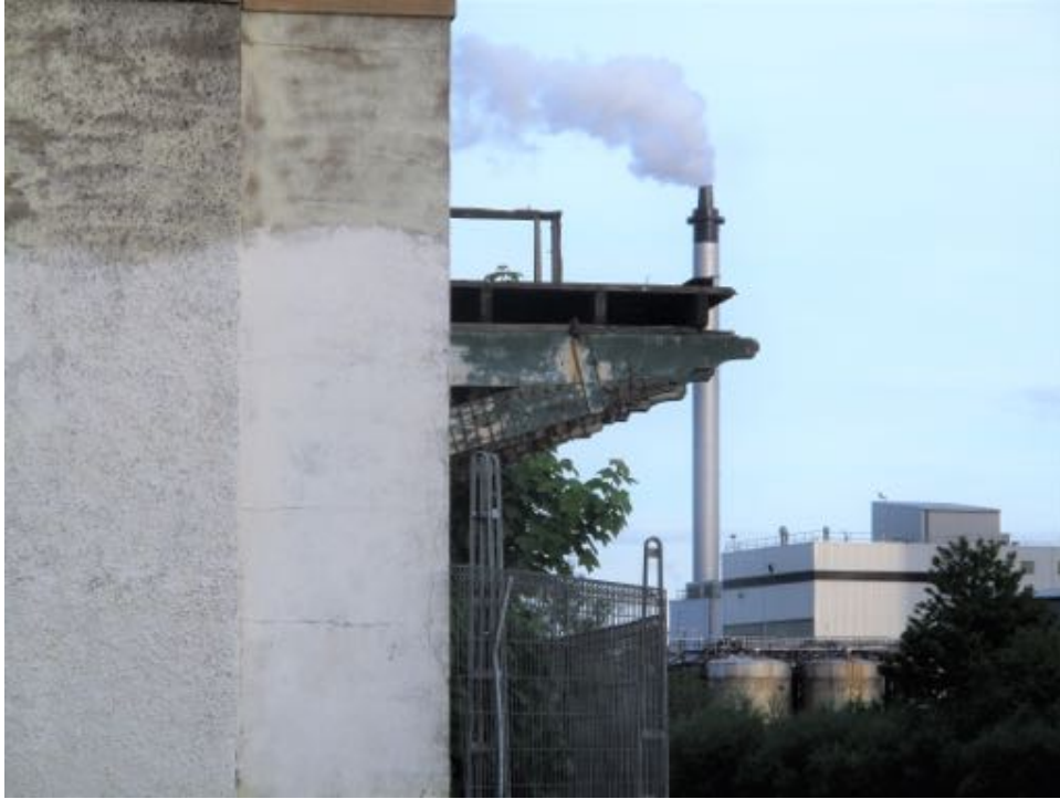
Photo 2 Wooden balcony with open space under floorboards
