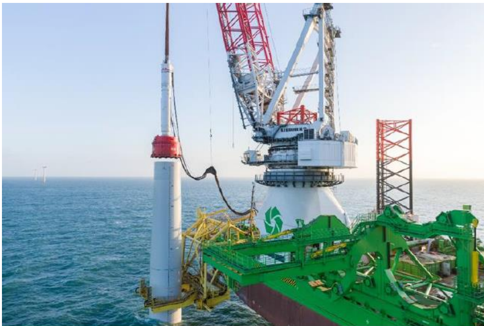
Figure 4-8: Example of the hammer being installed onto the top of the monopile.
