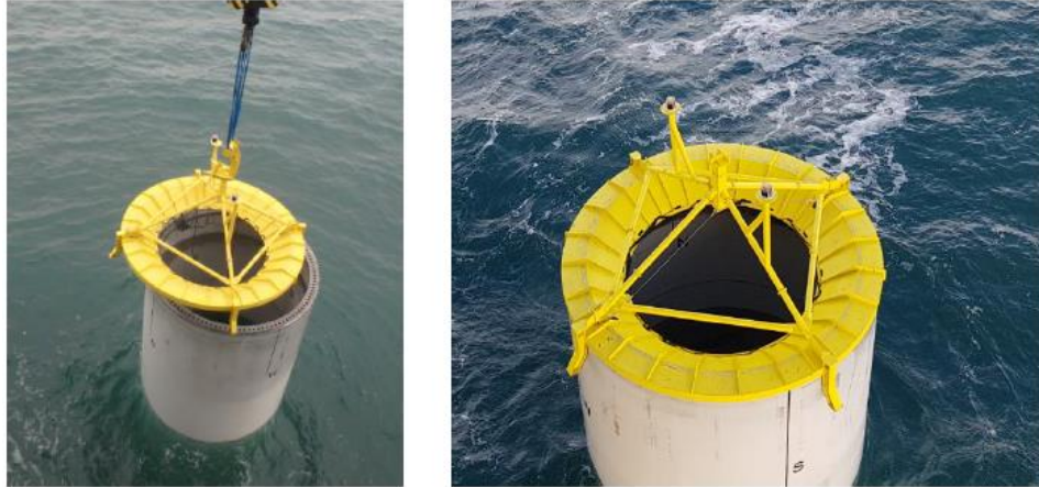
Figure 4-9: Example of a monopile cover installation.
