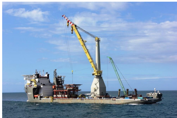
Figure 2-2: Example of pile installation vessels.
