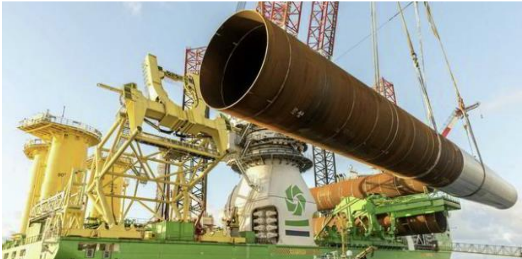
Figure 2-5: Example of a monopile being loaded up onto the installation vessel.
