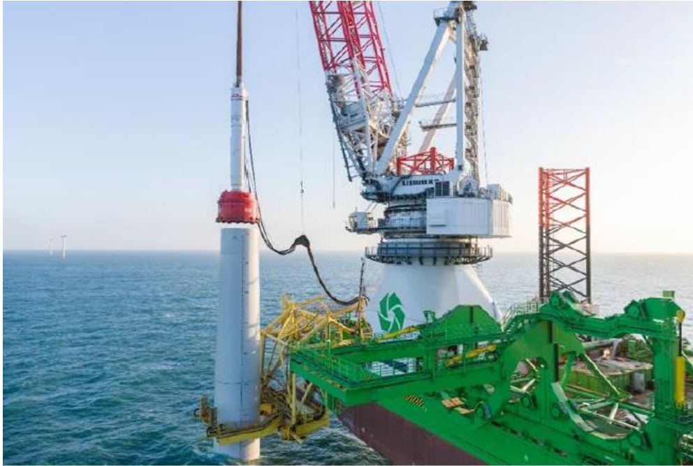
Figure 2-6: Example of the hammer being installed onto the top of the monopile.
