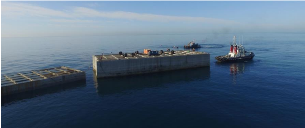
Figure 5-6 Caisson control platform and positioning equipment
