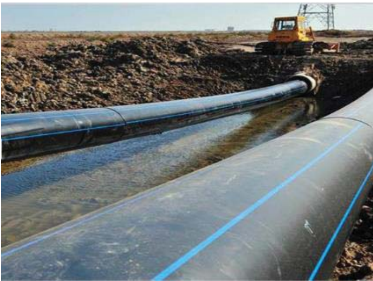
Figure 2.1: Trench Installation of Landfall HDPE Pipes into which Cables will be Pulled.
