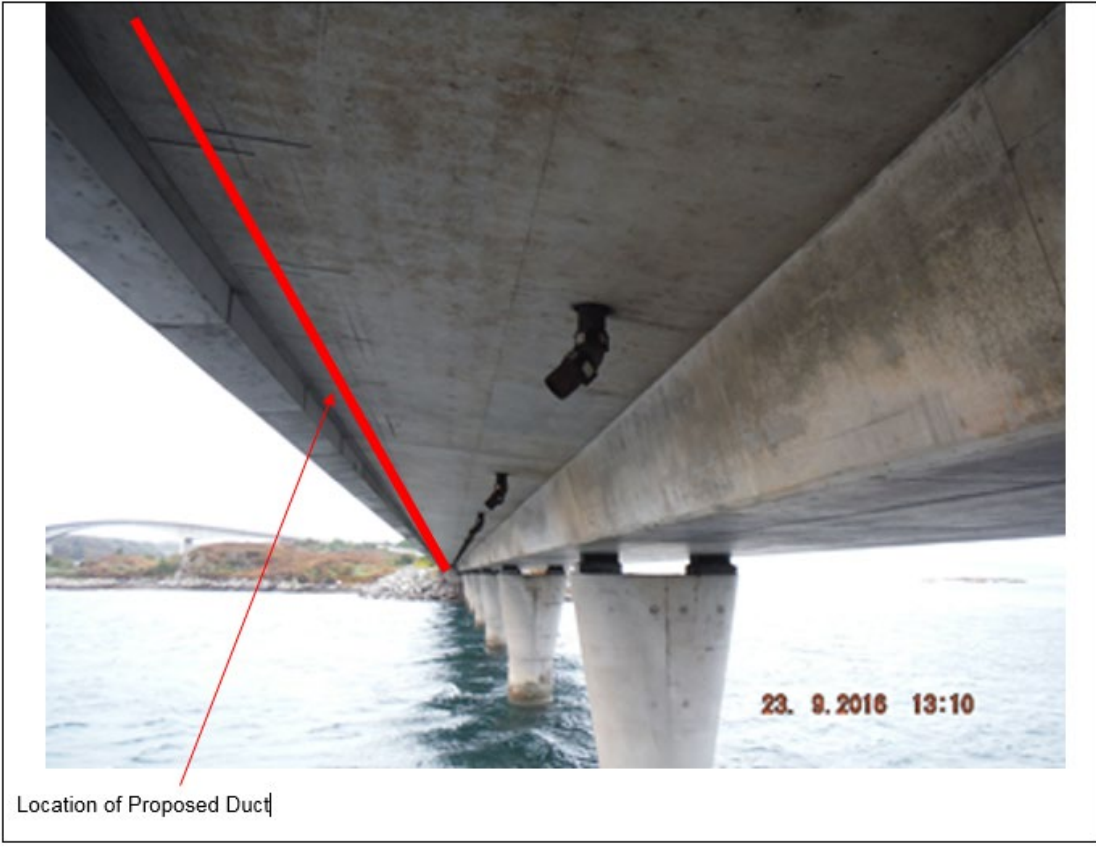
Photograph 1: Left hand Soffit of Carrick Bridge
